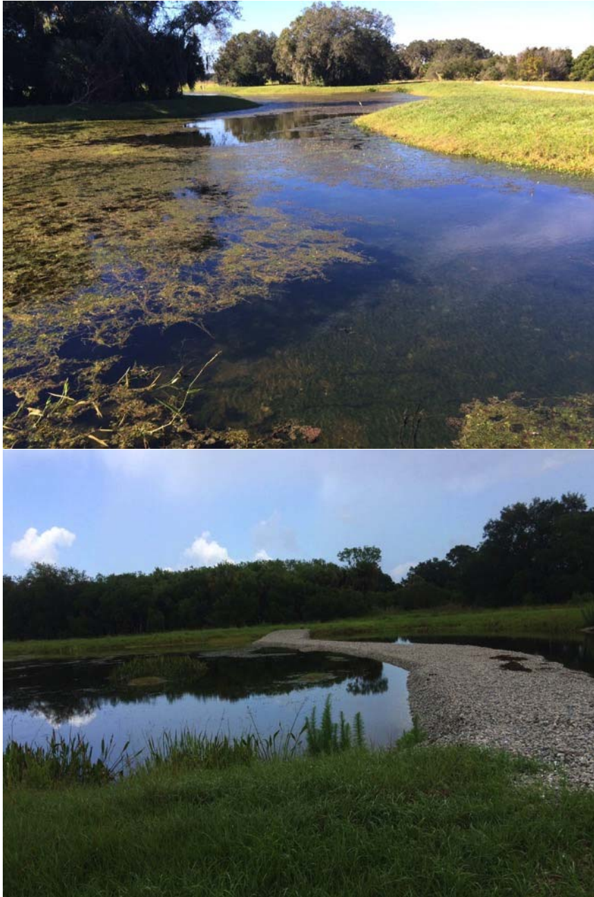
Figure 81. The eastern Grassy HWTT facility SAV pond (top), with the limerock bed (bottom) that was installed early in 2015.
