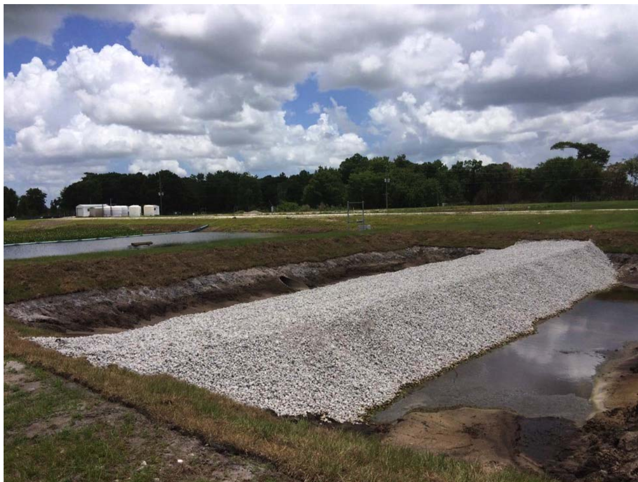
Figure 25. Outflow region limerock bed installed at the Mosquito Creek HWT in early 2015.
