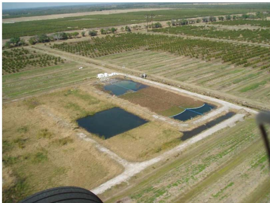
Figure 12. Aerial photo of the Ideal Grove HWTT facility.
