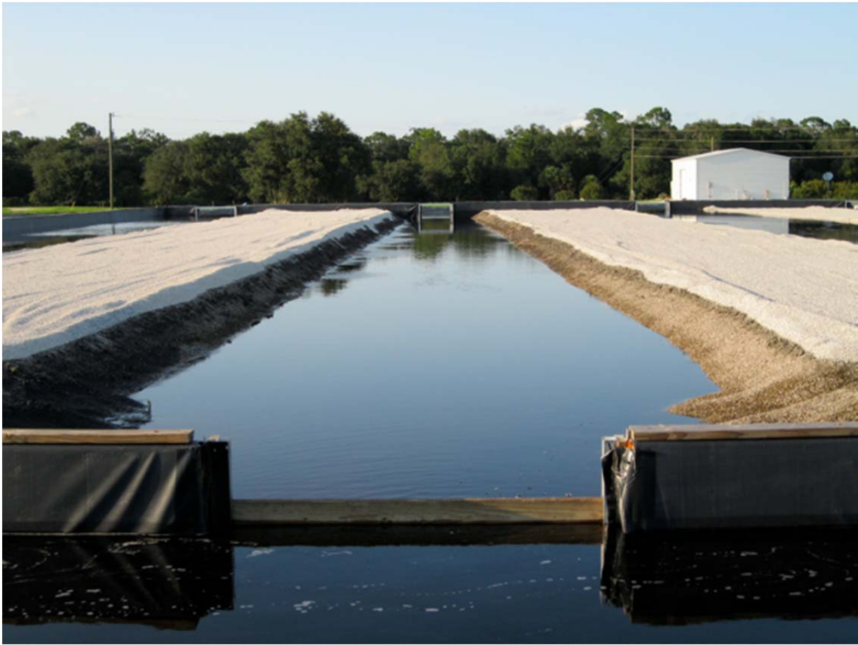
Figure 78. The limerock bed component of the Grassy HWTT facility.
