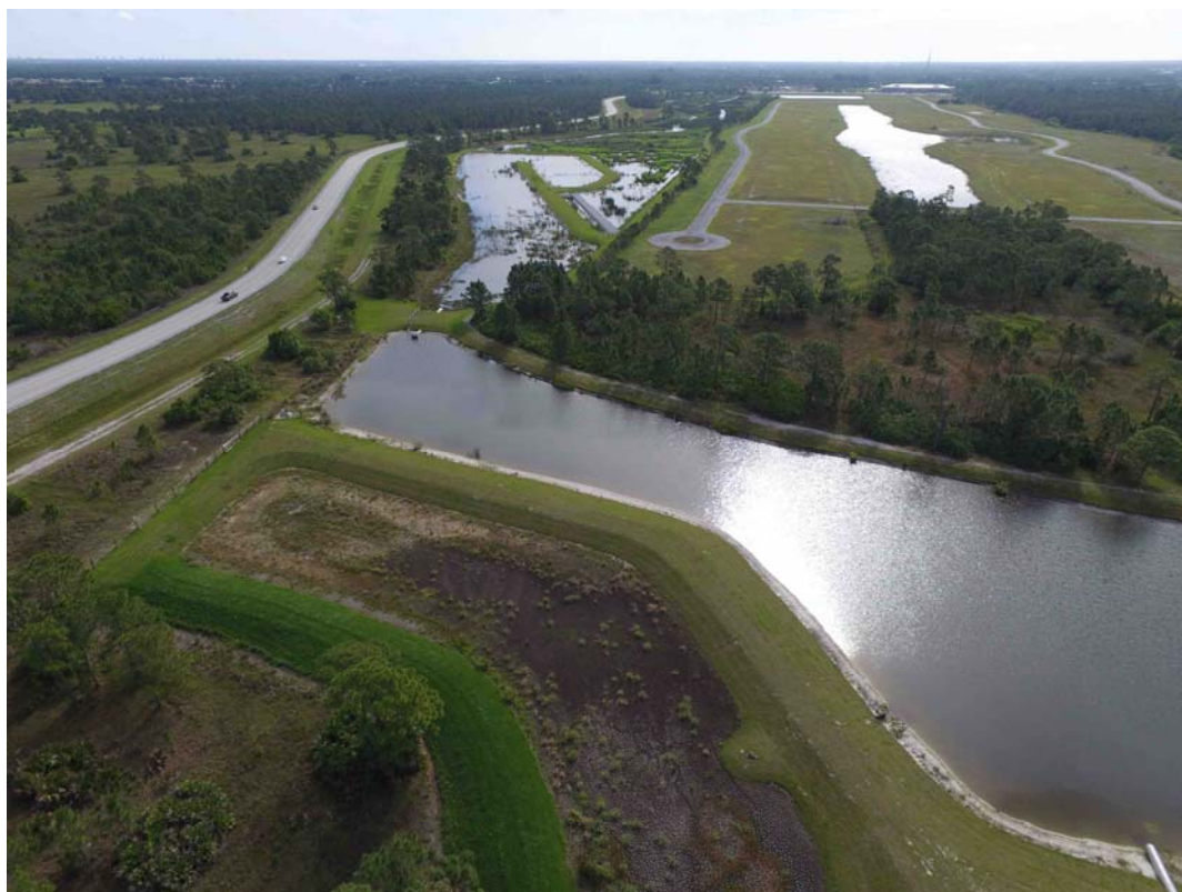
Figure 99. Aerial photo of the mid and outflow regions of the Bessey Creek HWTT system. Floc drying bed and settling ponds are shown in the foreground, and FAV and SAV ponds are visible in the top center of photo.
