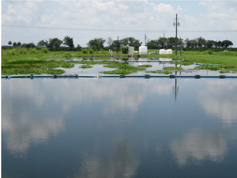
Figure 13. The outflow region of the Ideal Grove HWT facility.
