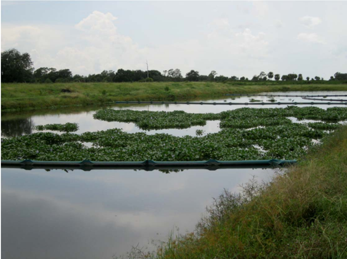
Figure 80. The eastern Grassy HWT facility FAV pond with three floating vegetation booms.
