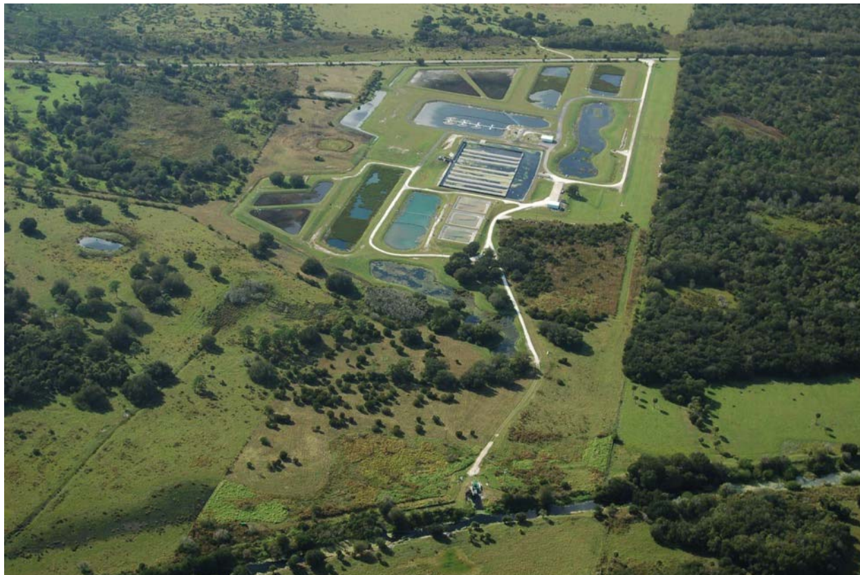
Figure 82. Photo of the final build-out of the Phase III Grassy Island HWT facility, completed in June 2013. Taylor Creek is at the bottom of the photo.
