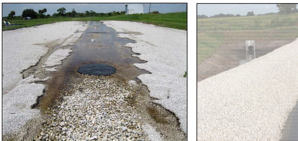
Figure 2. The inflow region (left) and outflow region (right) limerock beds at the Nubbin Slough HWTT facility.
