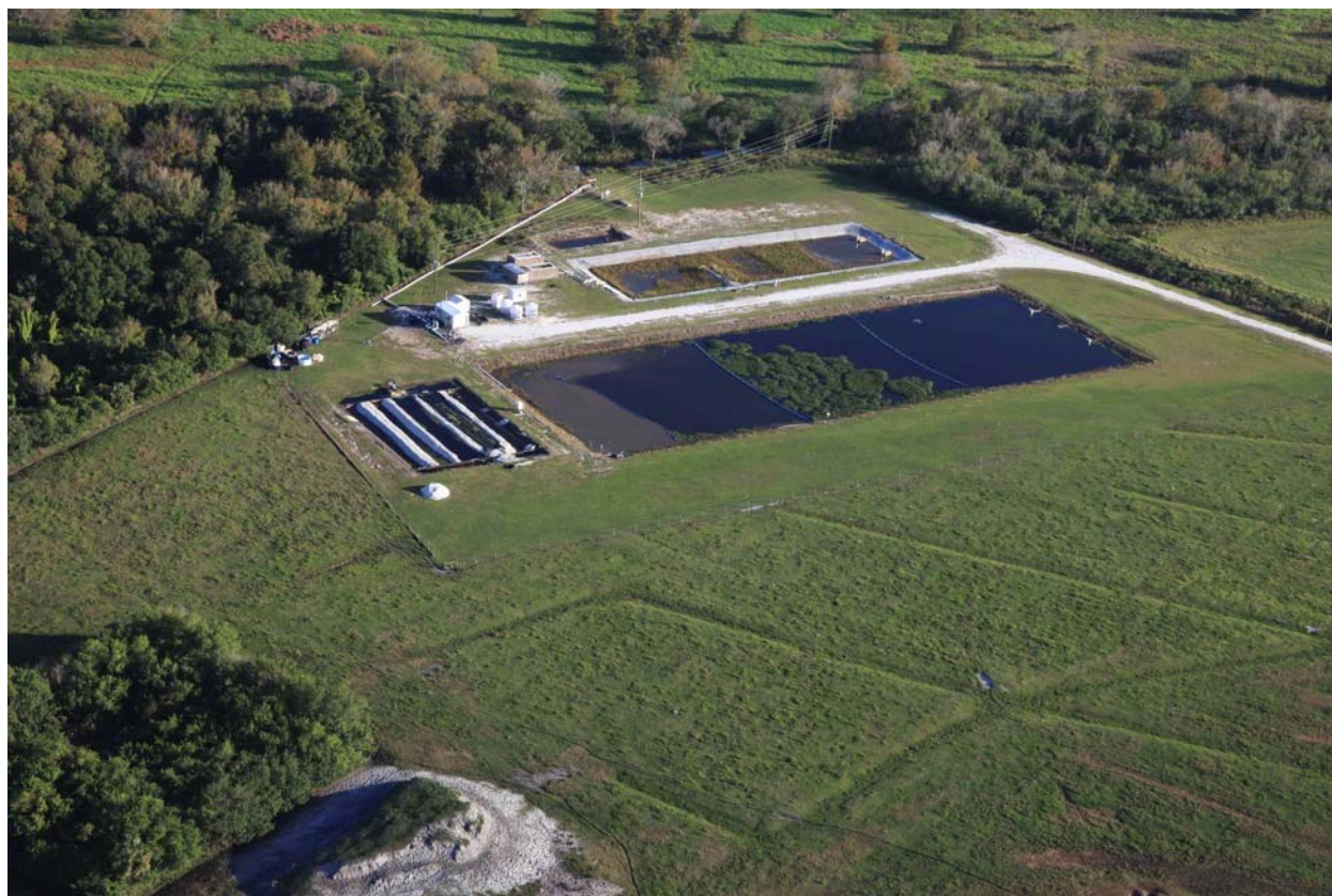
Figure 24. Aerial photo of the HWTT facilities at Mosquito Creek.
