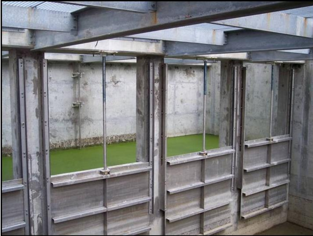
Figure 2-8. View of the Four Northern Downward Opening Weir Slide Gates Within the S-383 Distribution Box, with Gate Stem of Outlet Gate in Background.
