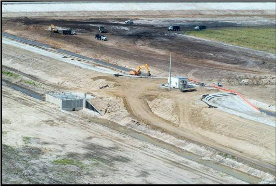
Figure 2-5. Structure S-383 during construction. Flow is from the reservoir on the right to the distribution box at the inlet to the treatment cell on the left.
