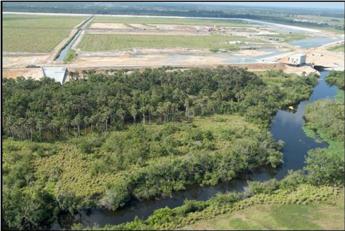
Figure 2-11. Photograph showing the emergency spillway in relation to the inflow pump station.
