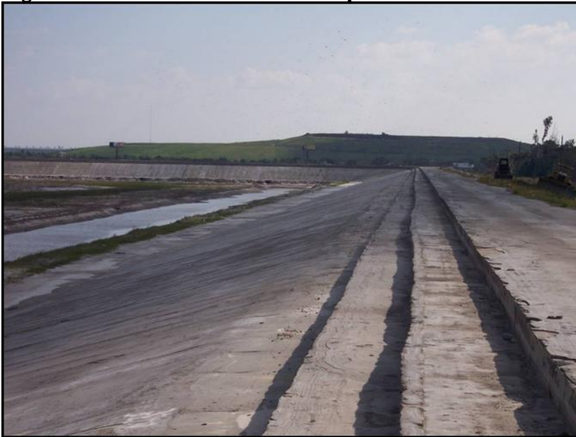
Figure 2-13. The armored inside slope of the reservoir cell showing the stepped top.
