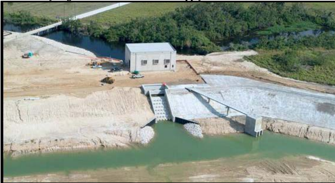
Figure 2-2. Photograph of reservoir side of S-382 showing the discharge drop structure and walkway to gate controls for the water supply release culvert.
