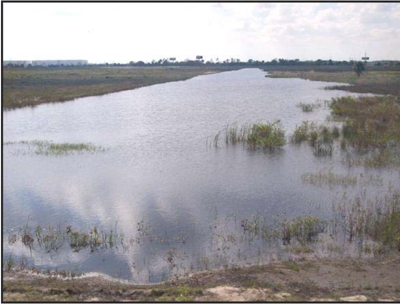
Figure 2-12. The deep zone trench in the middle of the treatment cell.
