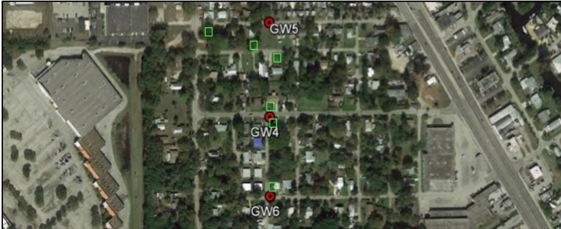
Figure 6. Groundwater monitoring wells (GW4-GW6) located near the “central drainage feature” in North Fort Myers, FL; the approximate location of some septic tank drainfields determined by the presence of mounding are indicated by the green squares. Not all drainfields in this area are represented in this map due to a lack of information.
