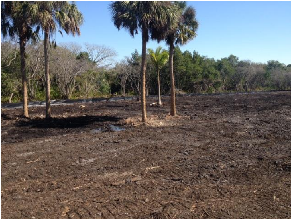
FIGURE 3: CITY OF FORT MYERS FORD STREET FILTER MARSH CONSTRUCTION
