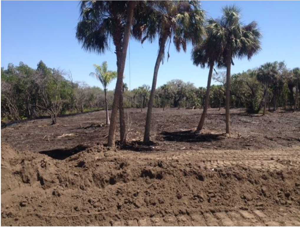
FIGURE B-5: CITY OF FORT MYERS FORD STREET FILTER MARSH CONSTRUCTION
