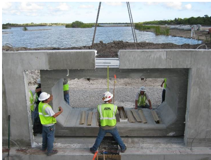
FIGURE 3: BREVARD COUNTY PINE ISLAND PROJECT UNDER CONSTRUCTION
