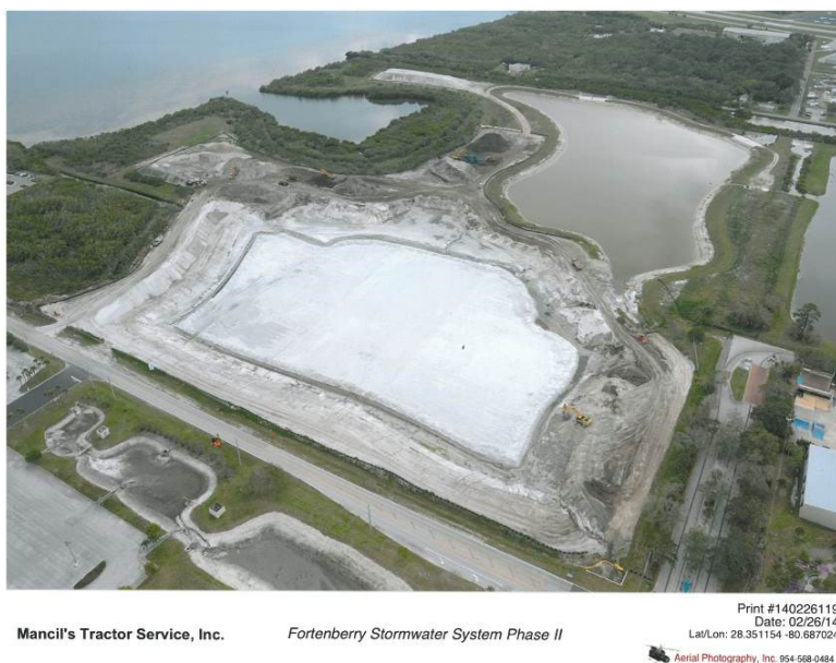
FIGURE 6: BREVARD COUNTY FORTENBERRY POND UNDER CONSTRUCTION
