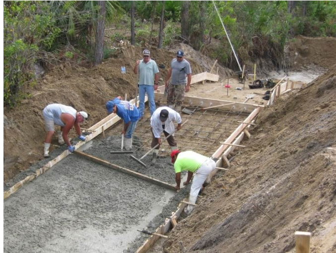
FIGURE 4: BREVARD COUNTY VALKARIA LAKES PROJECT UNDER CONSTRUCTION
