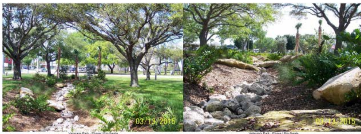
FIGURE 9: CITY OF FORT PIERCE VETERANS PARK PHASE I BIOSWALE
