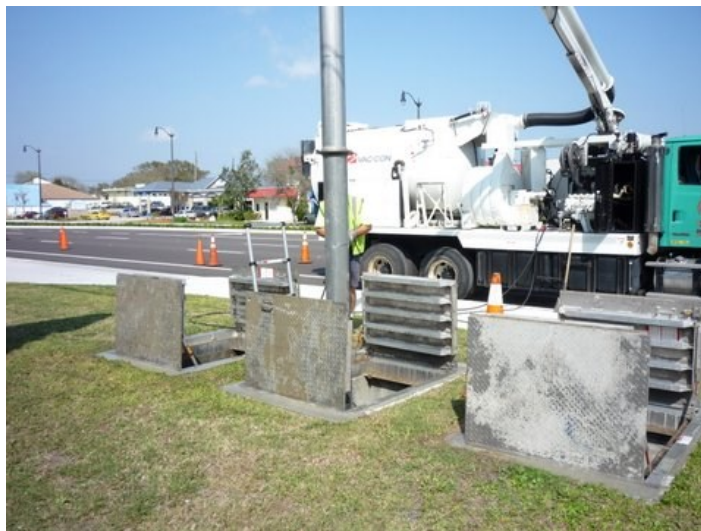
FIGURE 11: CITY OF ROCKLEDGE BAFFLE BOX CLEAN OUT
