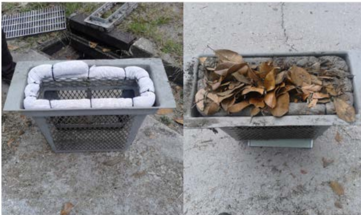
FIGURE 15: CITY OF TITUSVILLE INLET SKIMMER BOXES
