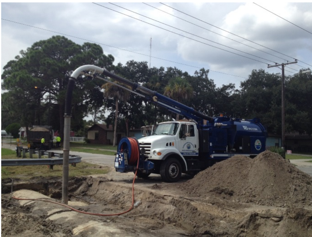
FIGURE 8: CITY OF TITUSVILLE STORMWATER PIPE CLEANING
