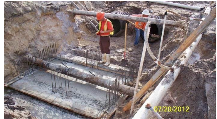
Satellite Beach Cassia Project Under Construction
