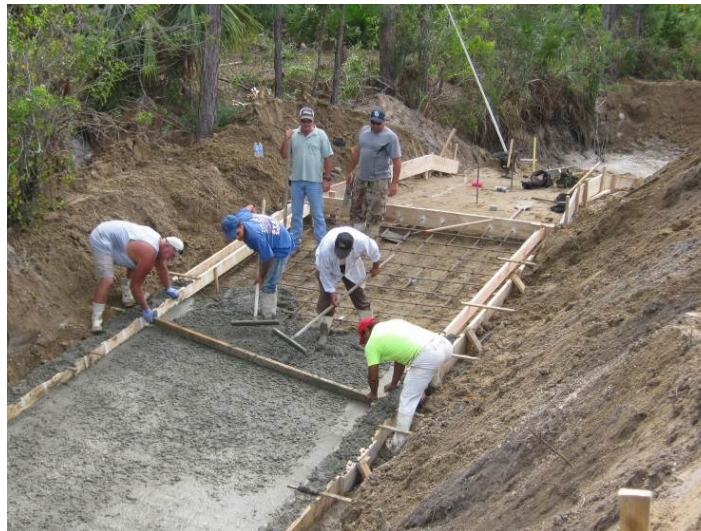
Brevard County Valkaria Lakes Project Under Construction
