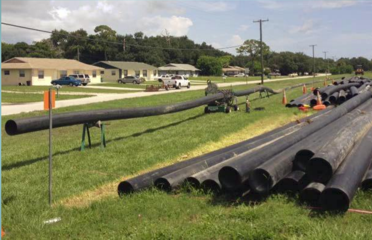
Fusing dredge pipe along Cherokee Avenue
