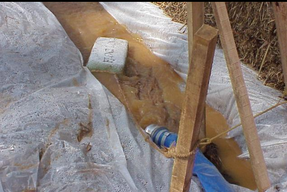
Simple Plastic-lined Ditch Treatment System
