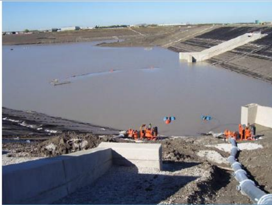
O'Hare South Basin - 75 million gallons in October 2008
