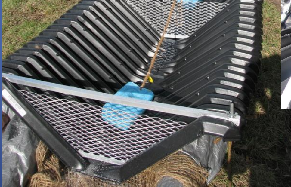
PAM Blend Floc Logs Installed In Smart Ditch
