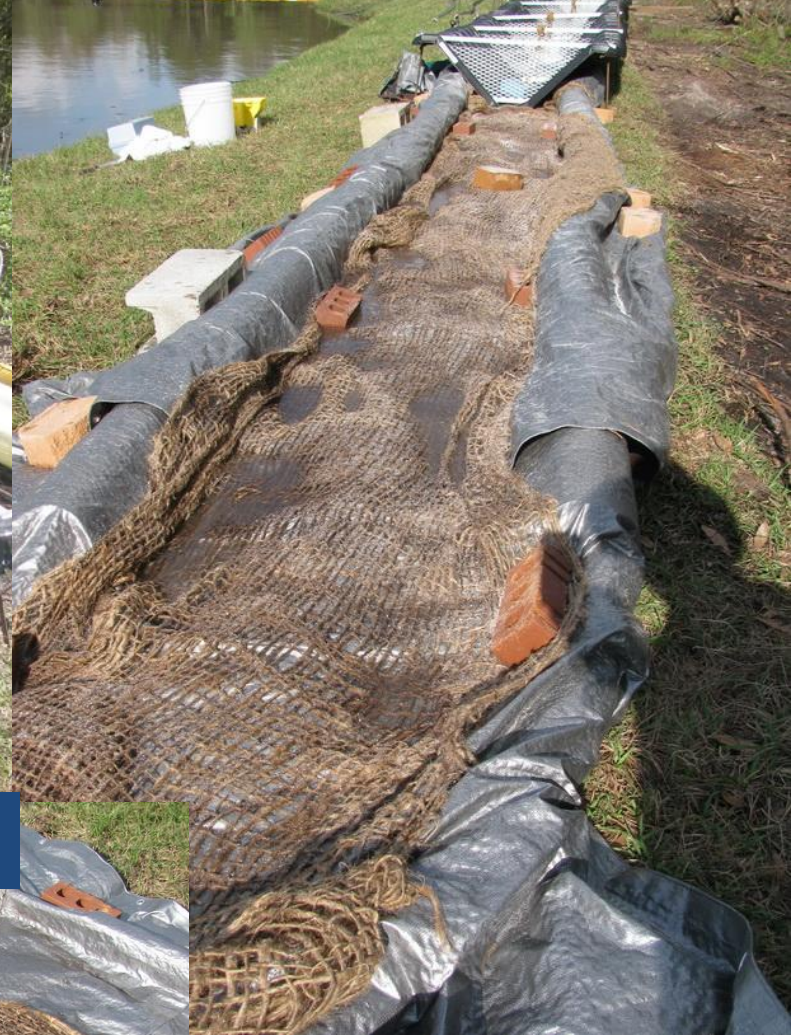
Smart Ditch Treatment System Set-up
