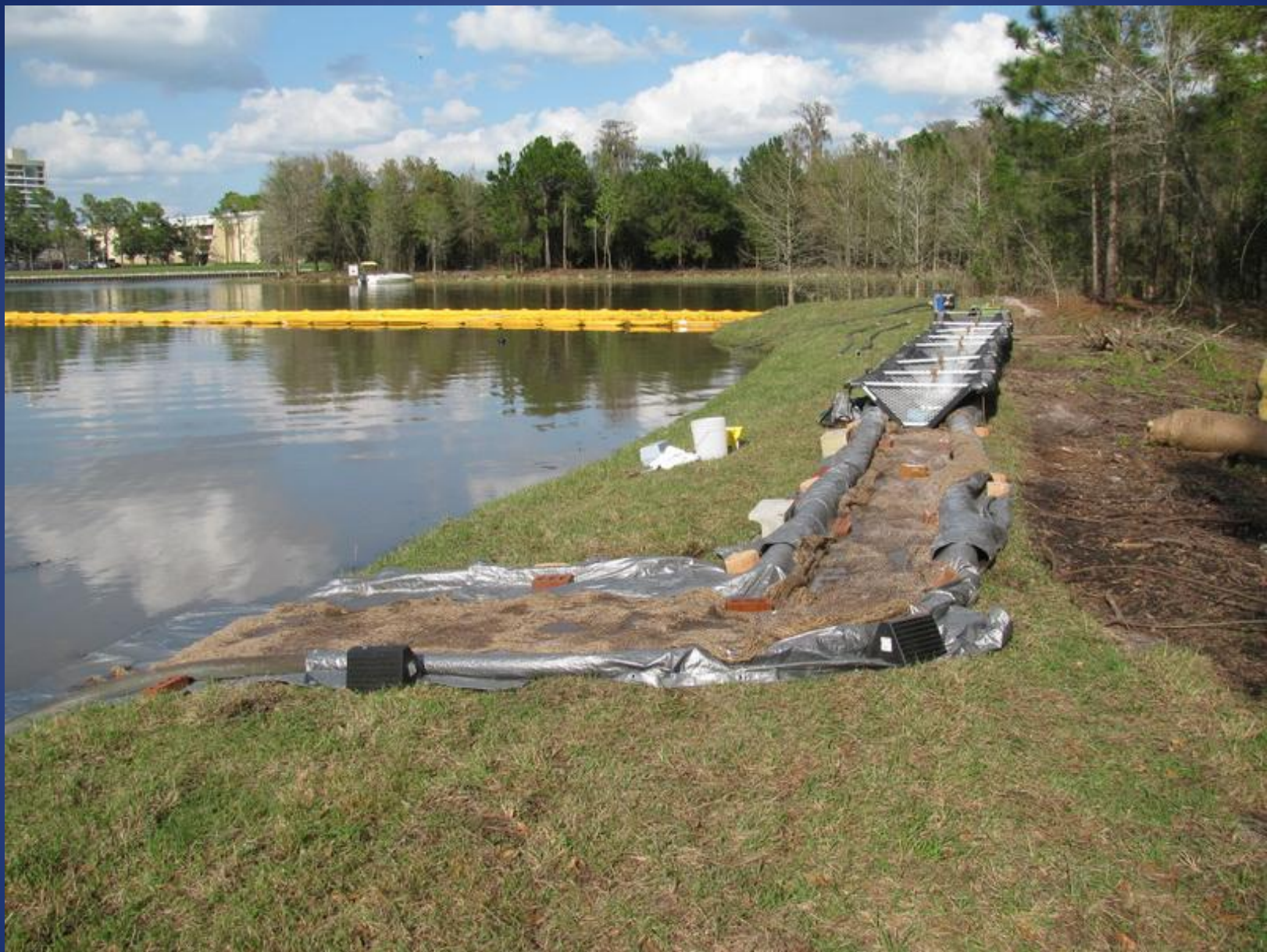
PAM Treatment System Set-up
