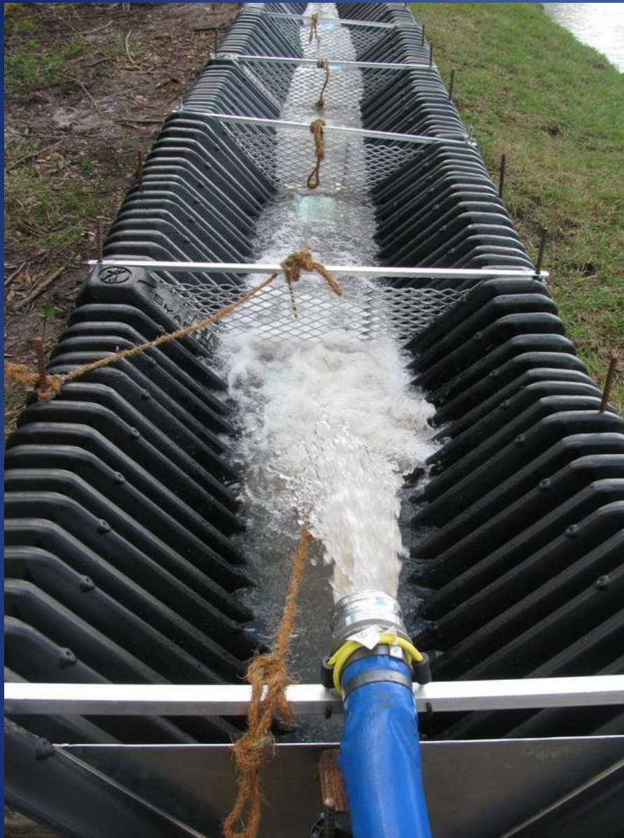
Pump Started, Floc Logs Dispersing PAM To Turbid Water
