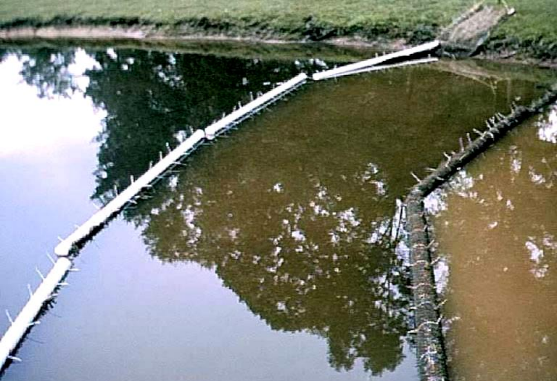
Particle Curtains For Floc Capture
