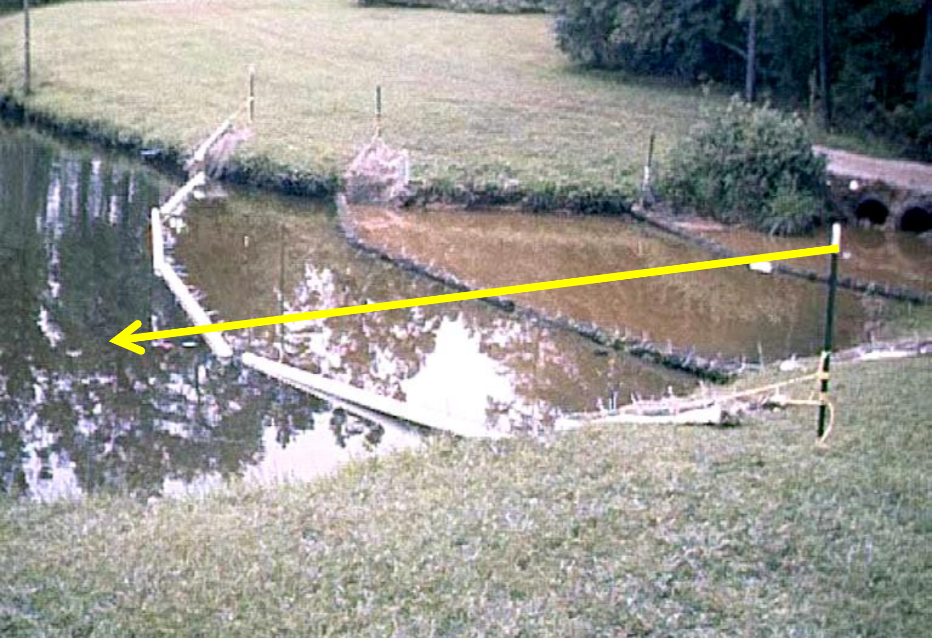
Particle Curtains For Floc Capture
