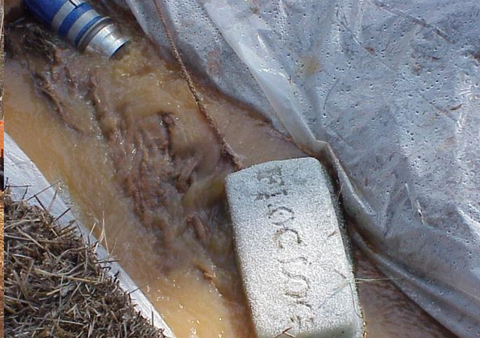
Simple Plastic-lined Ditch Treatment System
