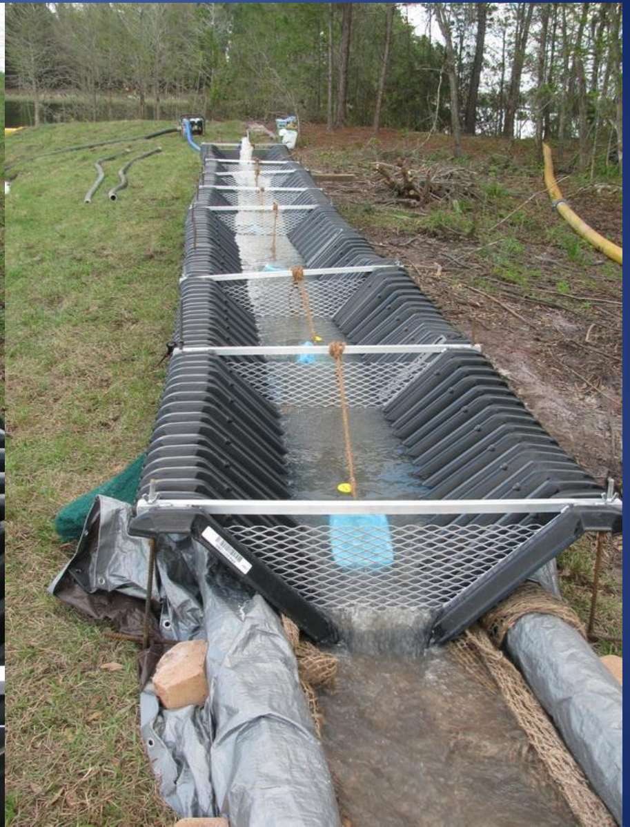
Pump Started, Floc Logs Dispersing PAM To Turbid Water
