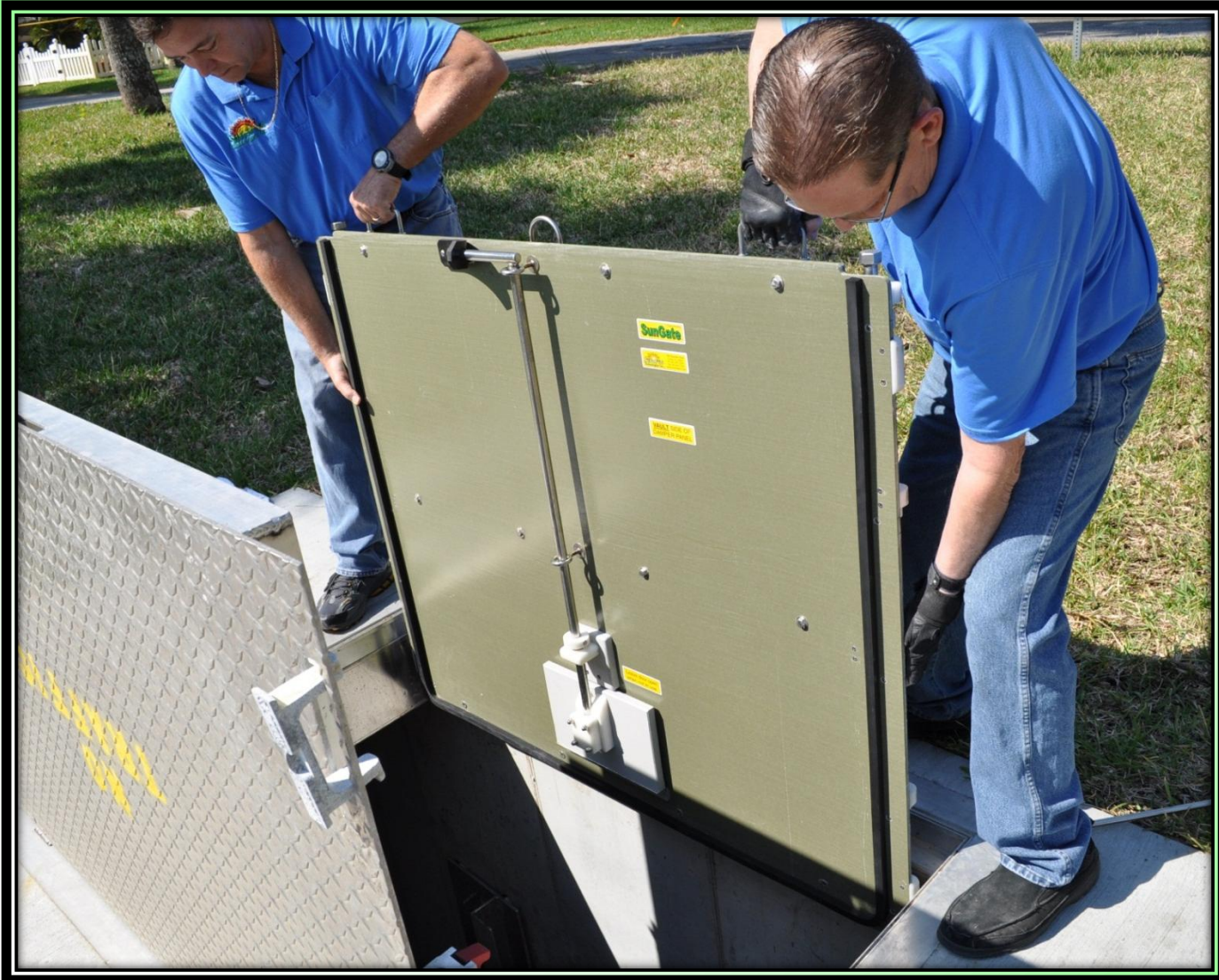
Lowering the SunGate through the hatch.
