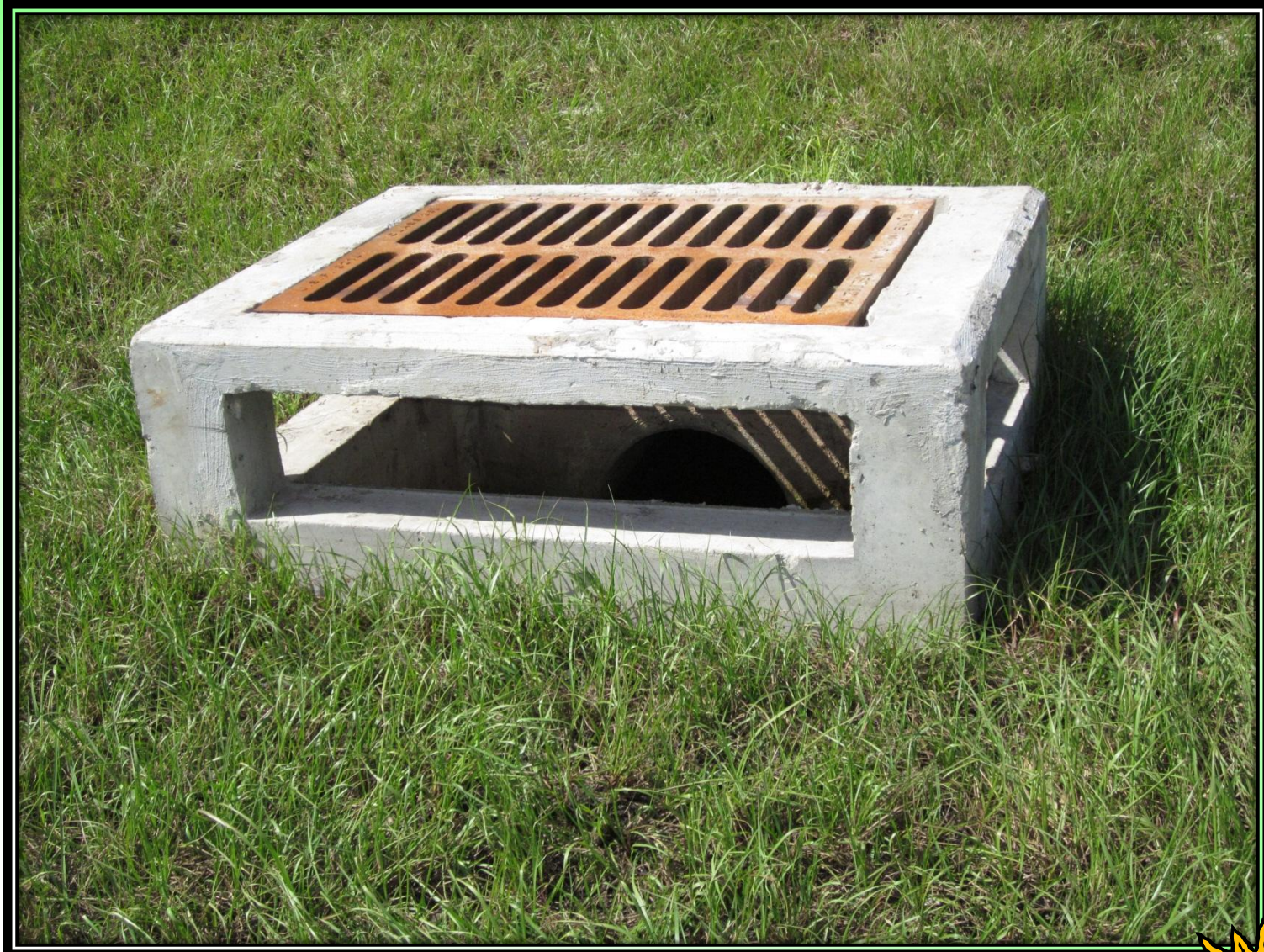
Outfall structure in detention area.
