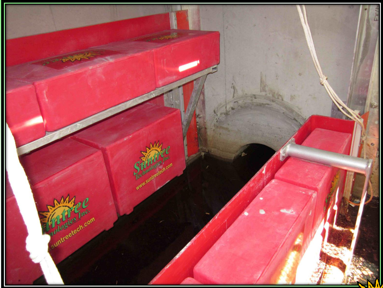
View of SkimBoss Diversion Weir
