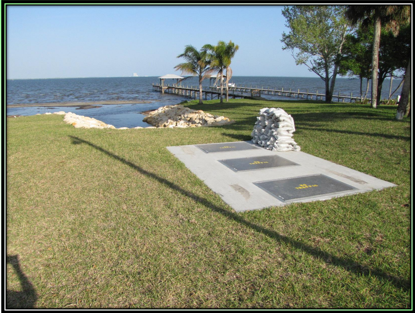
The finished installation.
