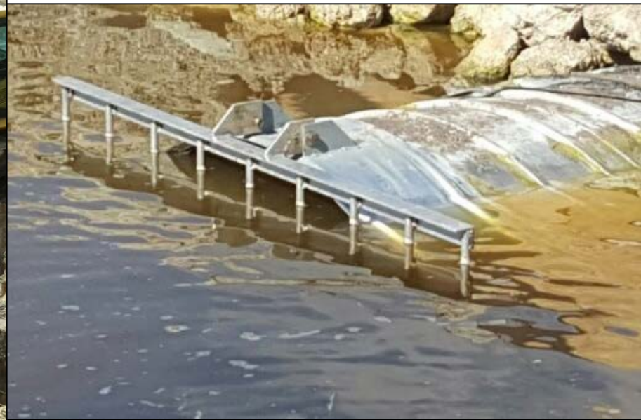
OK-7: Lock 7 Bypass Culvert System Project
