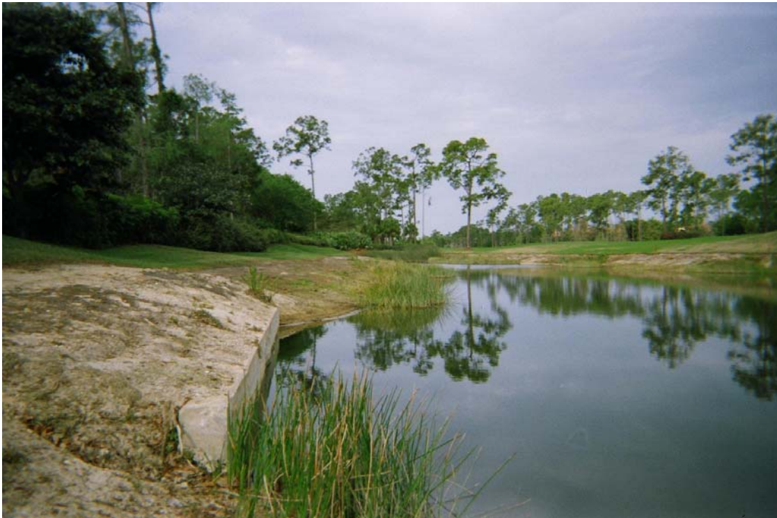
View west at headwall on outfall culvert located at south end of project and just upstream of outfall weir (see below).
