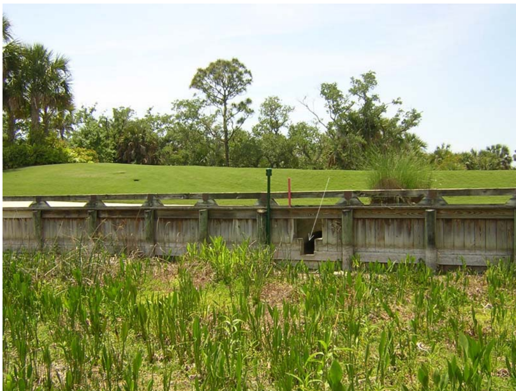
View Water Control Structure SW-LA12. Structure is located at arrow in wooden retaining wall.
