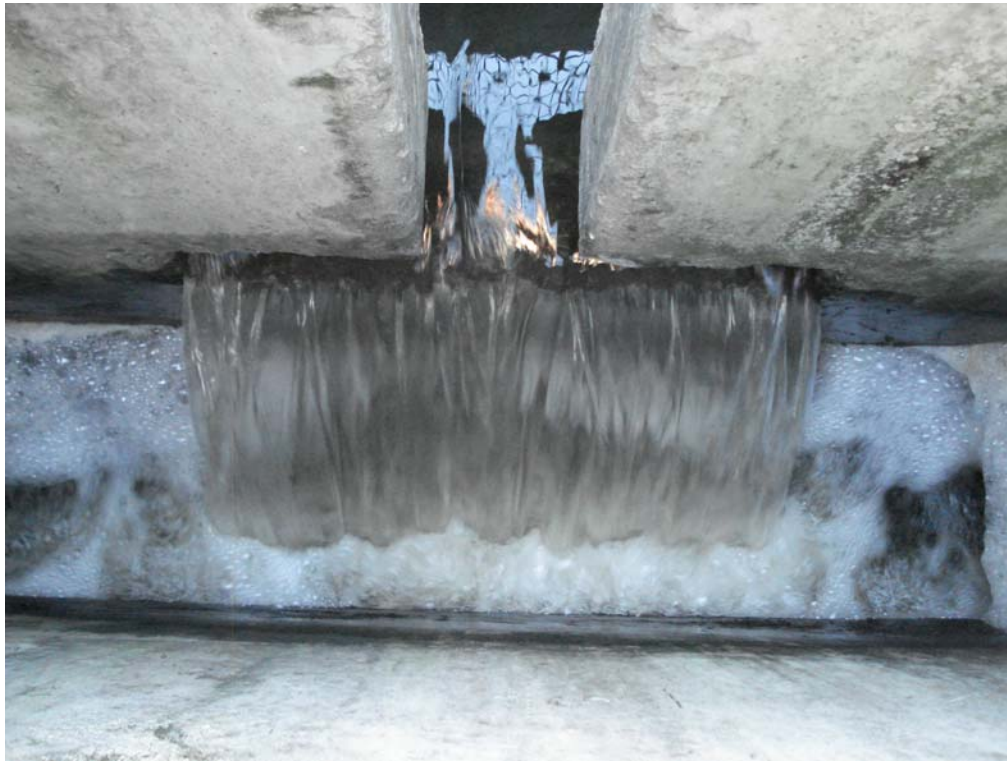
Water Control Structure WS-1. Photo taken September 13, 2008. View inside inlet at flow over control weir.
