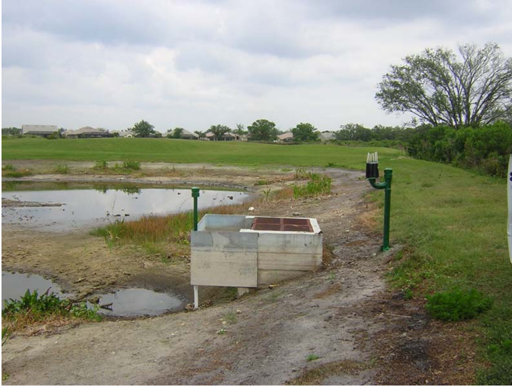
Water Control Structure WV-L4 – View east.
