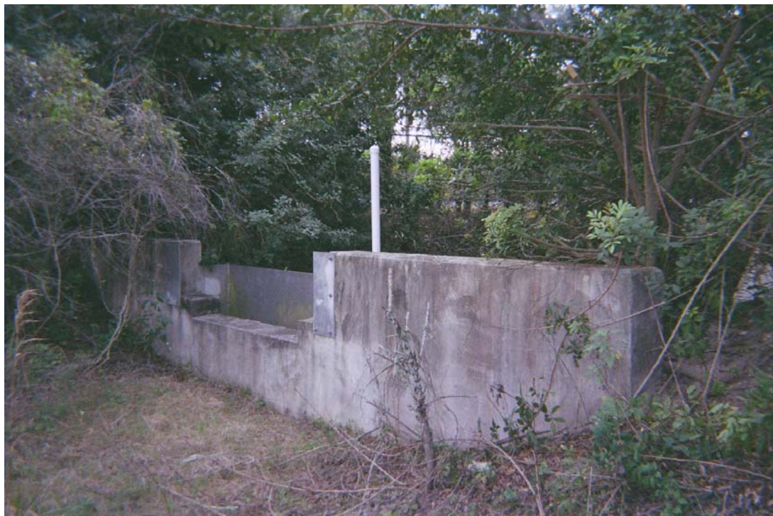
View southeast at outfall weir structure. Photo taken March 23, 2008.
