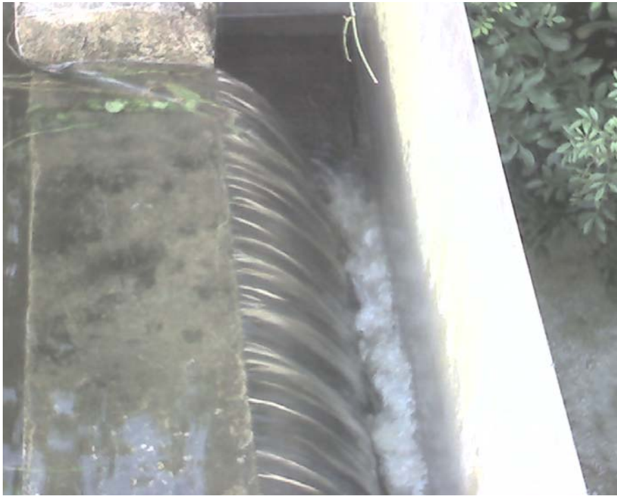
Photo shows first documented flow since January 2007 at WT-2 outfall following heavy rainfall from Tropical Storm Fay. Photo taken August 20, 2008.
