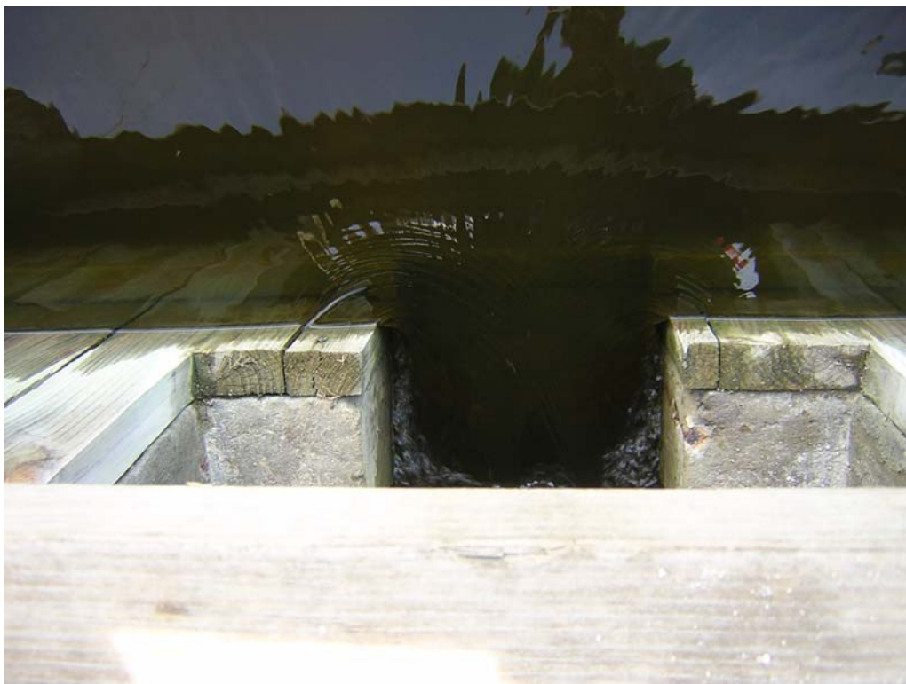
View vertically down at flow over Water Control Structure SW-LA12. Photo taken July 17, 2008. See previous page E-3A (top) for horizontal photo of structure.
