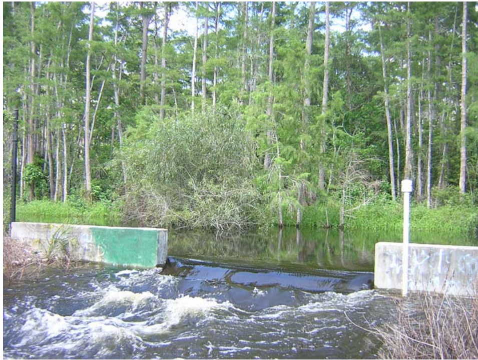
View northeast across L-28 weir. Photo taken July 17, 2008. Refer to graph page C-12 to see stage of approximate elevation 14.8' that corresponds to this photo.
