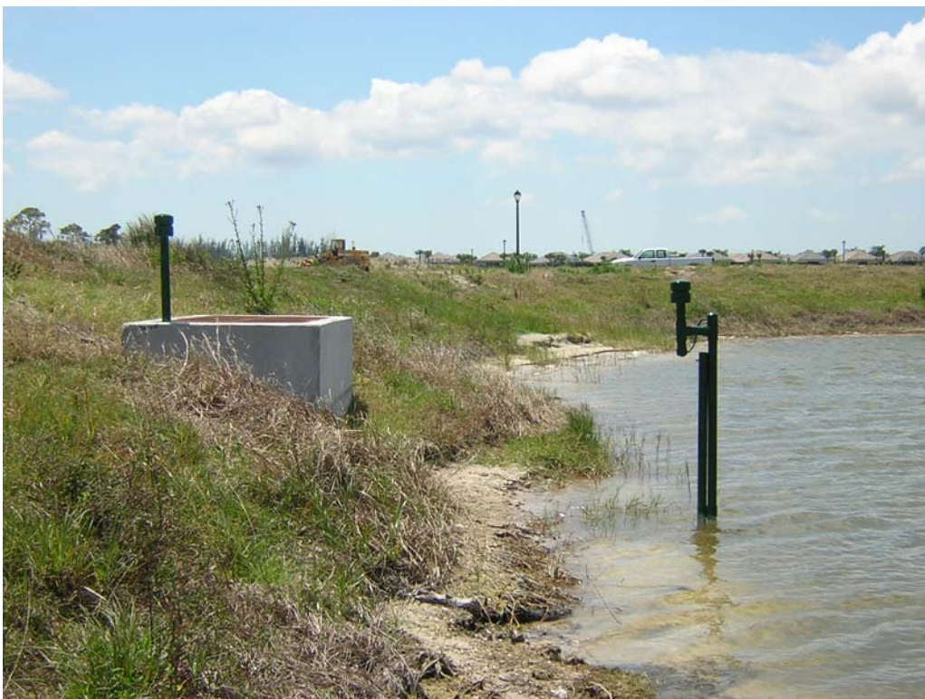
View south at structure WS-3 and recorders.
