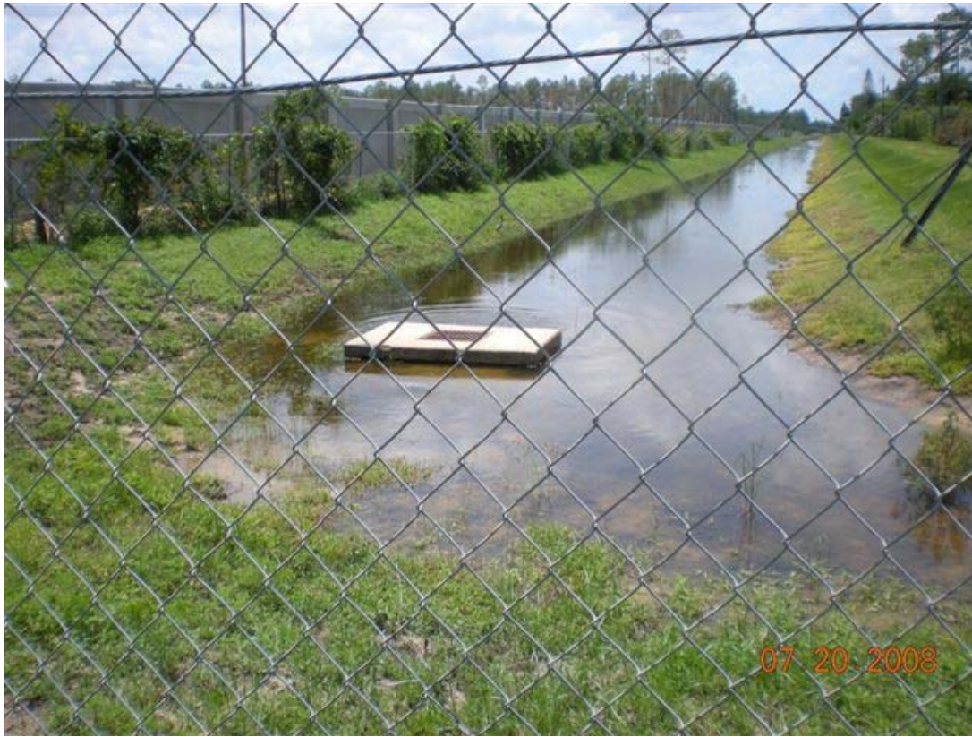
Mediterra outfall to south. Note flow ripples in swale downstream of submerged notched structure. Photo taken July 21, 2008.
