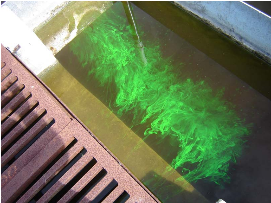
Water Control Structure WV-L4 – View northwest. Photo taken July 11, 2008 Slow velocity, under submerged condition was measured by movement of dye.
