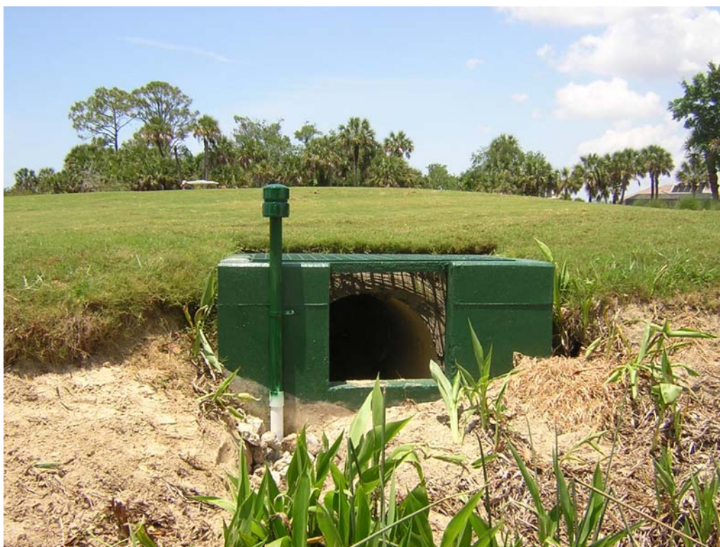
View Water Control Structure SW-LA8. Upstream stage recorder is at left of inlet face. Photos taken May 1, 2007.
