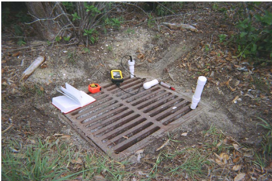
Outfall weir (beneath grate). Downloading data from stage recorders inside inlet.
