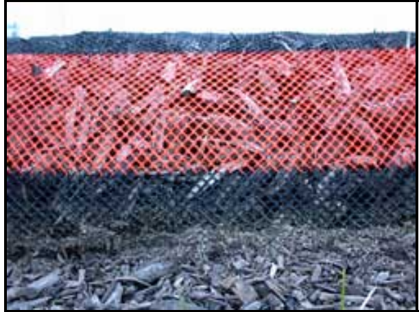
Detail of compost-filled mesh sock (Source: Filtrexx, 2006)
