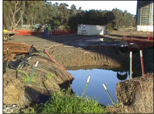
Sediment Trap (Source: http://www.mnerosion.org )
