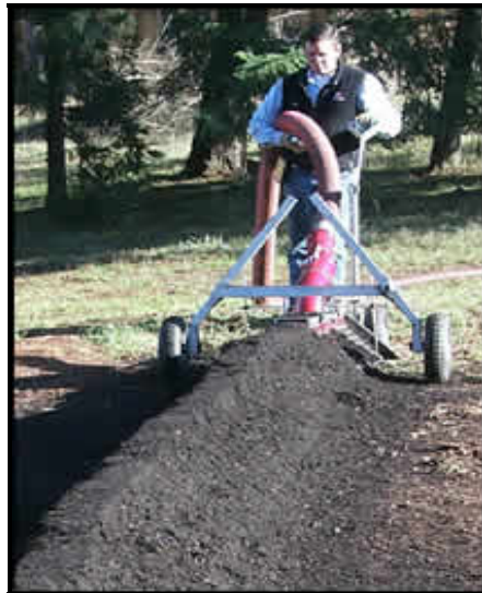
Installation of compost berm (Source: Rexius, 2006)
