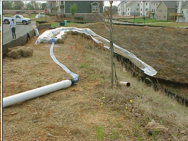
Figure 3: The water was pumped through the pipe mixers and down a jute lined ditch.
