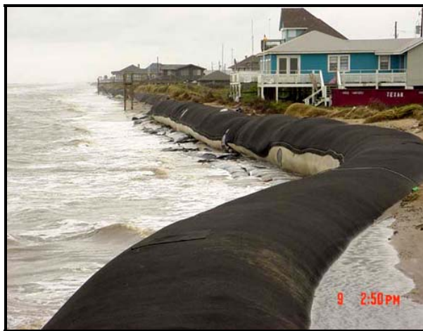
Sandsack, sand-filled tubular geotextile (Source: Surfrider Foundation, 2006)
