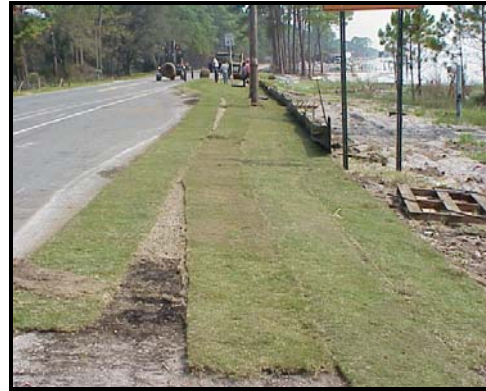
Final placement of sod
