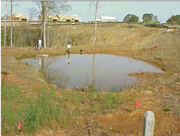
Figure 2: The water was pumped out of the sediment pond.
