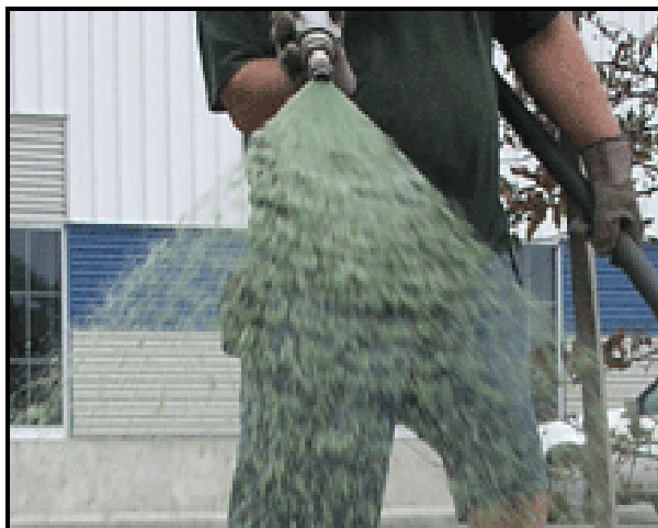
Hydraulic mulch sprayer (Source: Price and Company, 2006) Dyed hydraulic mulch (Source: Terra-Mulch, 2006)
