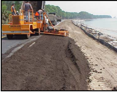
Placement of compost mulch layer
