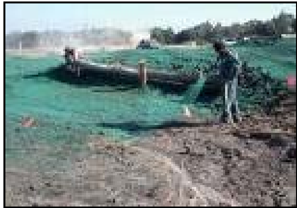
Hand application of hydroseed on construction sites (Source: RMB Craftscapes Ltd, 2006)
