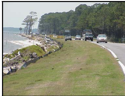
Roadway and shoulder successfully protected
