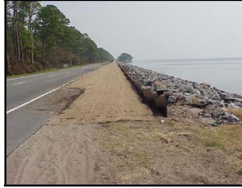
Placement of jute fiber erosion control blanket
