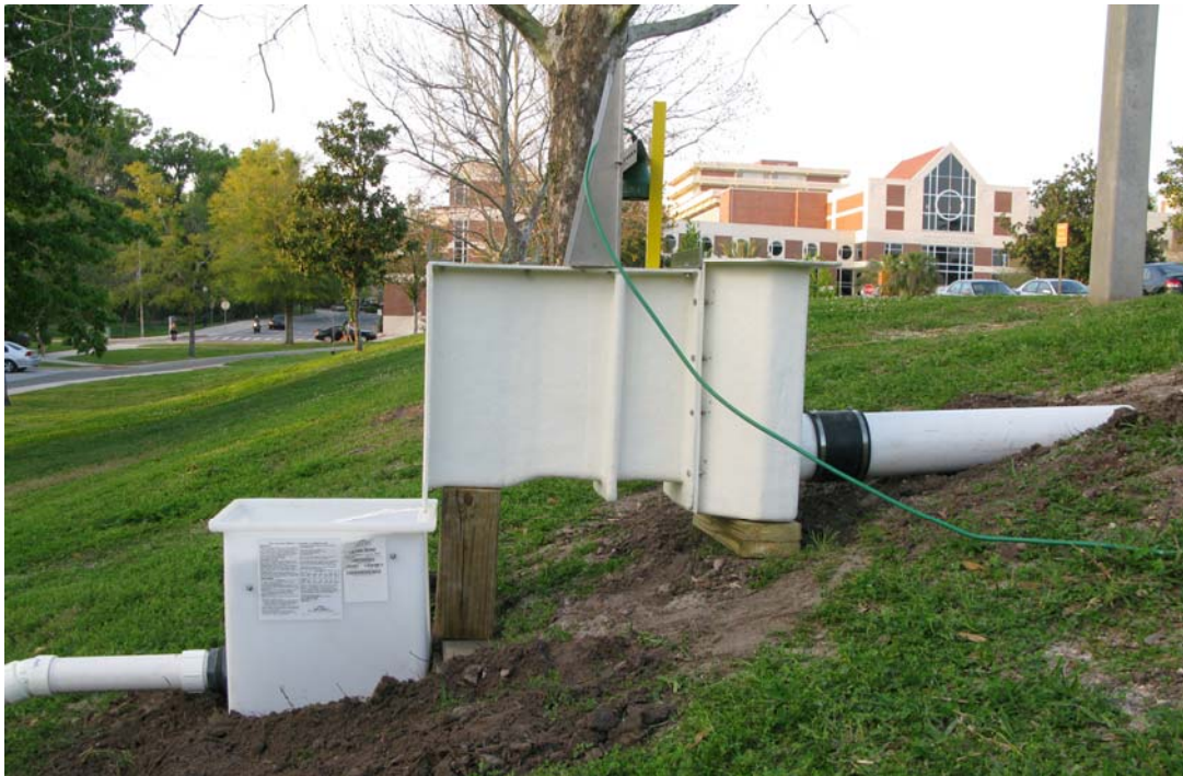
Figure 7 Monitoring system as installed. The flow rate measurement system: Parshall flume and drop box.
