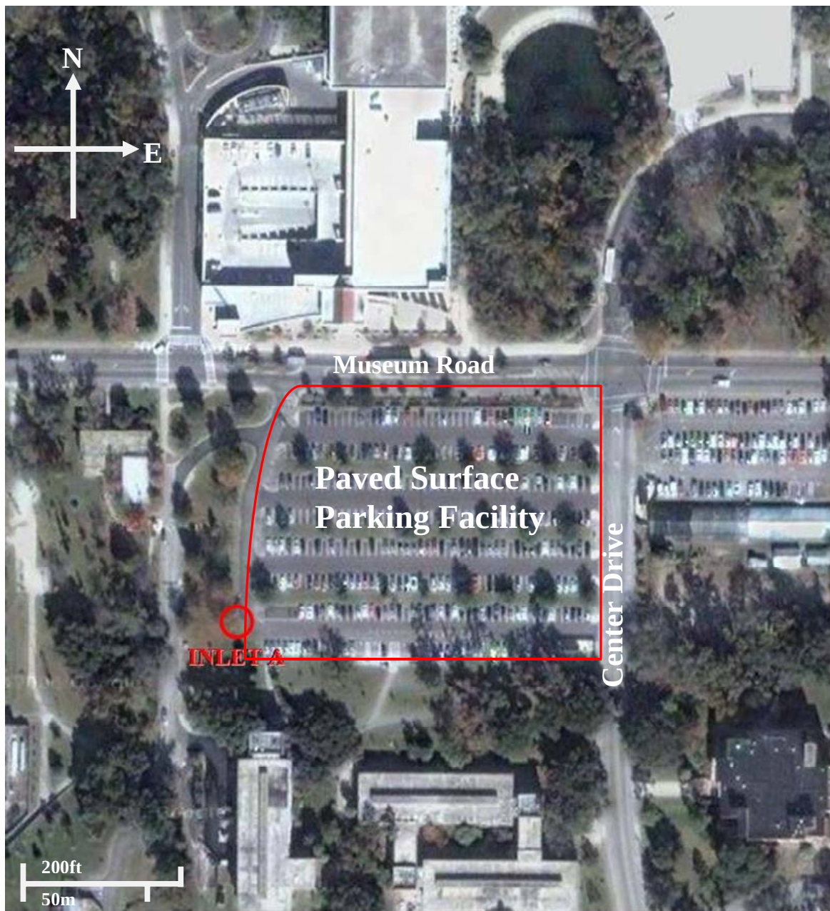
Figure 1 University of Florida Reitz Union paved surface parking facility in Gainesville, FL. Particular of the monitored inlet.
