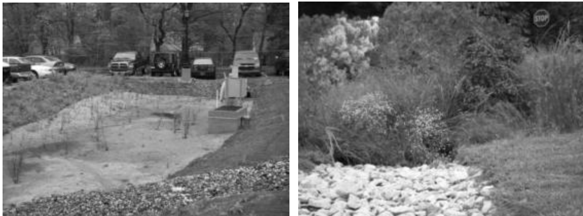
a. Newly Planted (left) and Well-Established (right) Bioinfiltration Basins.
