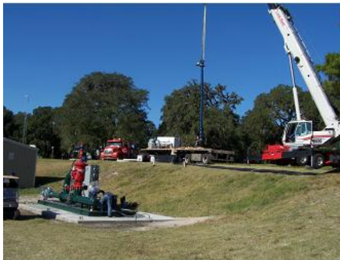
VERTICAL TURBINE PUMPS INSTALLATION
