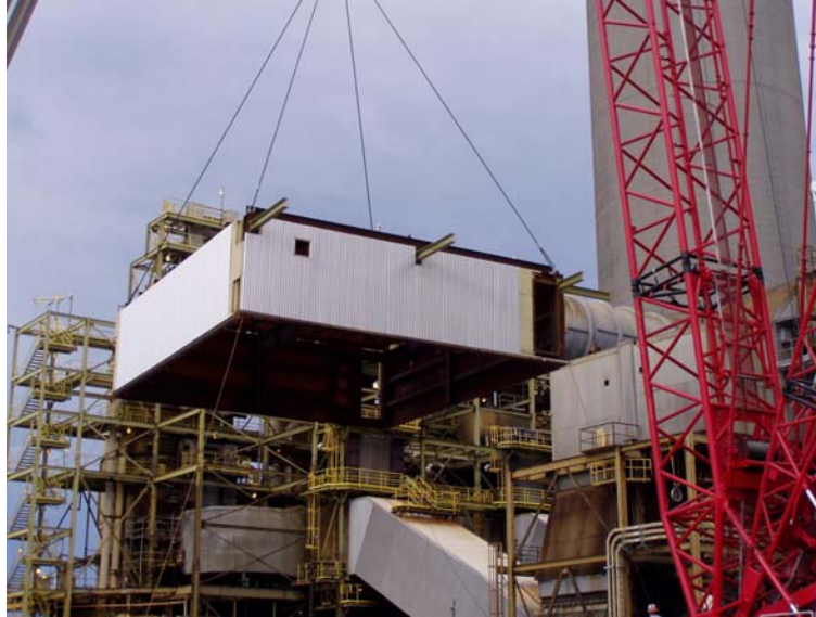
FIGURE 4: INSTALLATION OF SCR BOX
