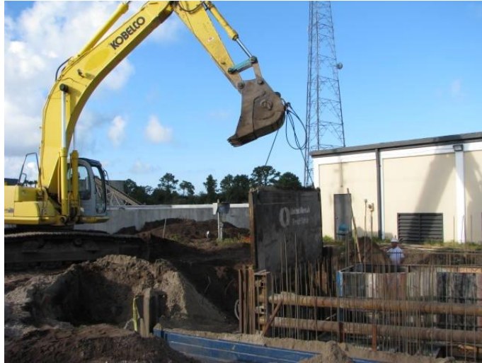
EXTRACTION OF TEMPORARY SHEET PILING FROM THE NEW BAR SCREEN STRUCTURE AREA
