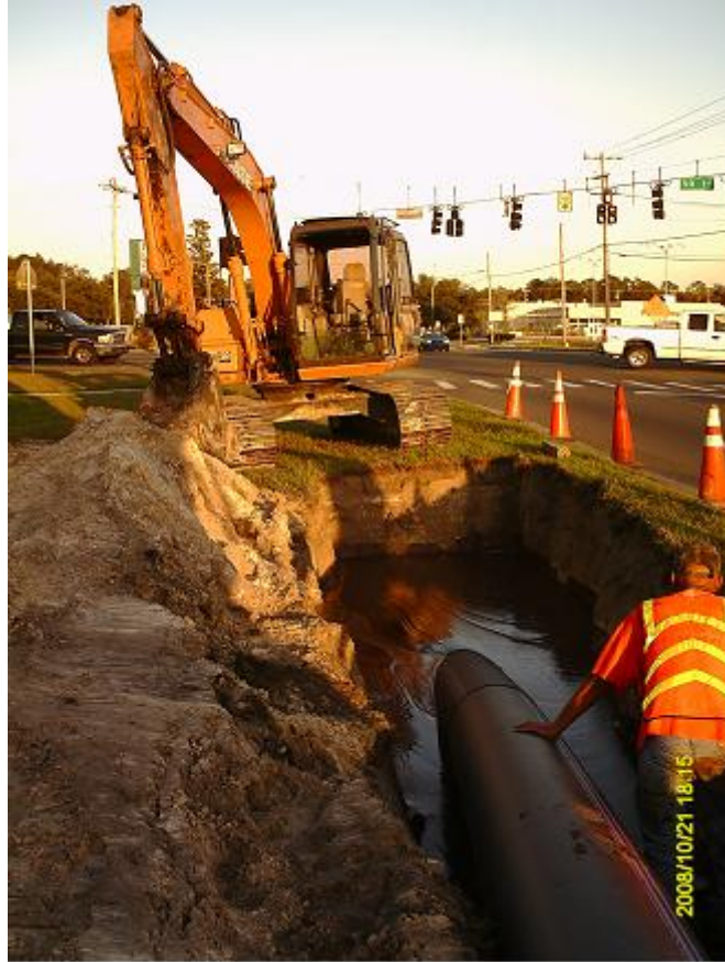
18-INCH HIGH DENSITY POLYETHYLENE (HDPE) DIRECTIONAL BORE UNDER STATE ROAD 19
