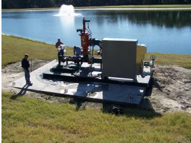
NEW RECLAIMED WATER PACKAGE PUMP SKID INSTALLATION
