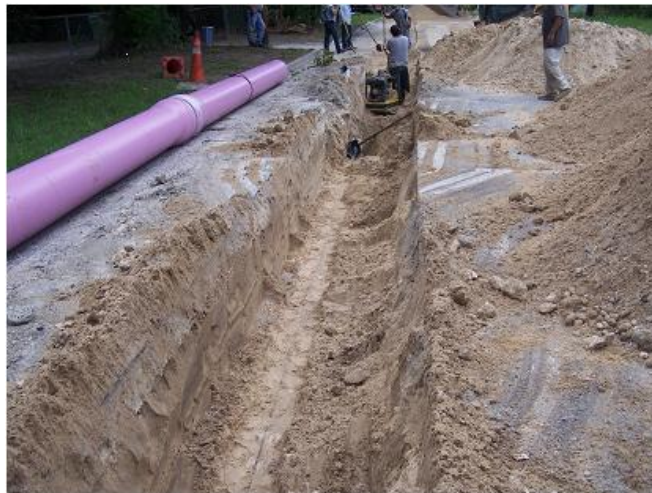
INSTALLATION OF 16-INCH PVC RECLAIMED WATER MAIN
