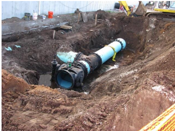
INSTALLATION OF 24" INFLUENT BY-PASS PIPING ON WEST SIDE OF CHLORINE CONTACT TANKS
