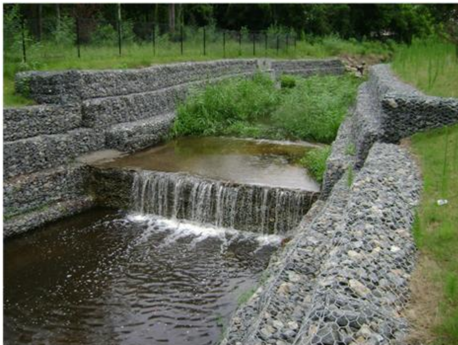
CITY OF JACKSONVILLE REGIONAL STORMWATER FACILITY OUTFALL
