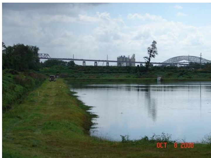
UPPER DEER CREEK REGIONAL STORMWATER FACILITY
