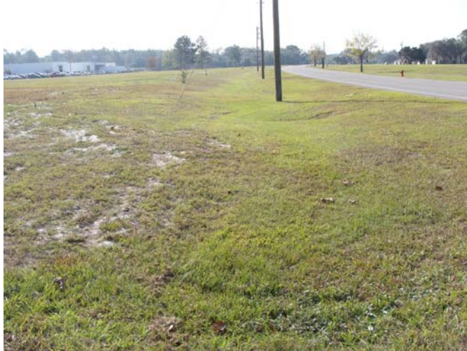
AVENUE A SWALE FROM JACKSONVILLE STREET
