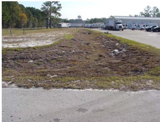
J6 OFFICE SWALE REPAIR
