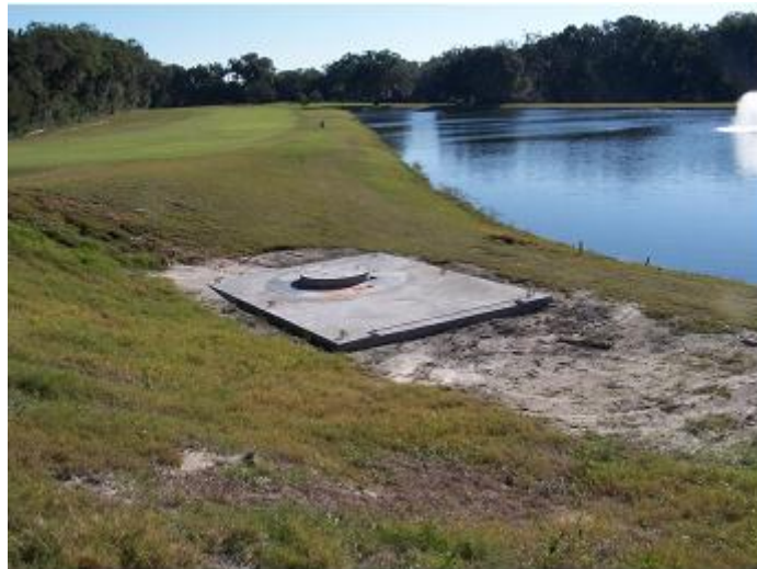
NEW RECLAIMED WATER PUMPING STATION BUILDING FOUNDATION
