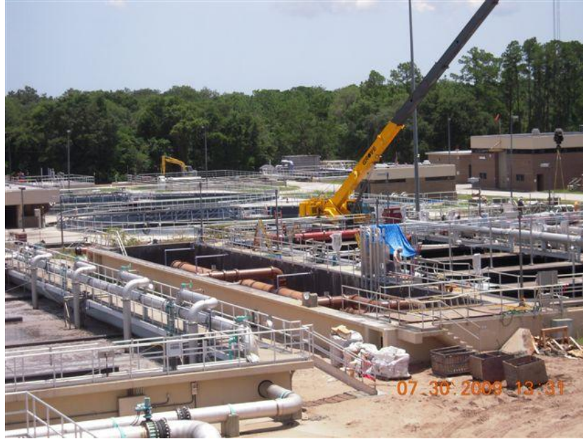
FIGURE 10: JEA ARLINGTON EAST WWTF CONSTRUCTION PROJECT
