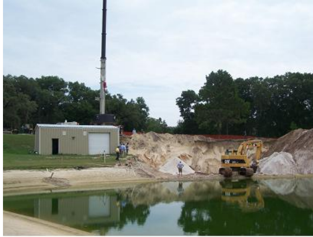
PRE-CAST WET WELL INSTALLATION AT GOLF COURSE RECLAIMED WATER HOLDING POND
