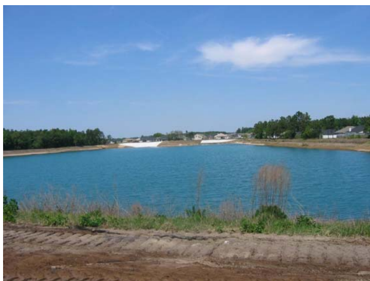
SANDALWOOD CANAL BORROW PIT STORMWATER FACILITY
