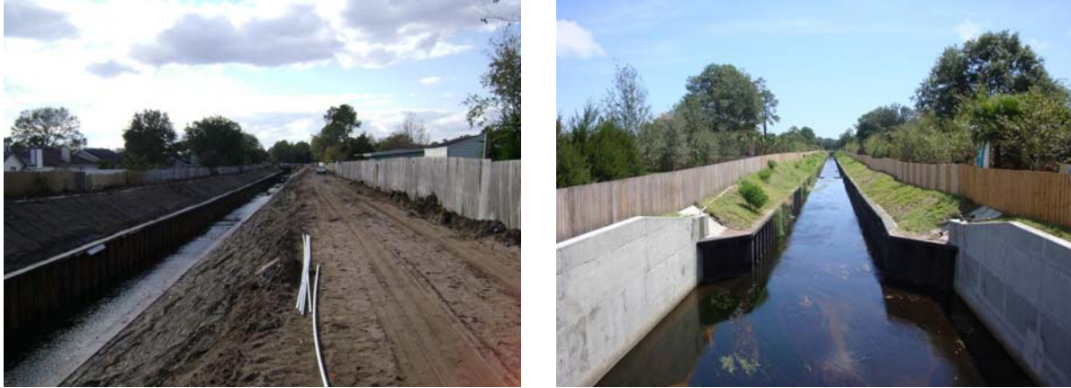
FIGURE 16: CITY OF JACKSONVILLE SANDALWOOD CANAL UNDER CONSTRUCTION AND COMPLETED
