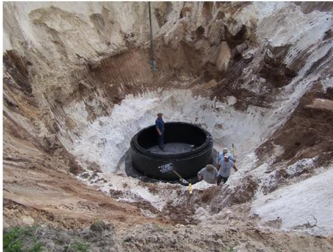
NEW PRE-CAST WET WELL INSTALLATION
