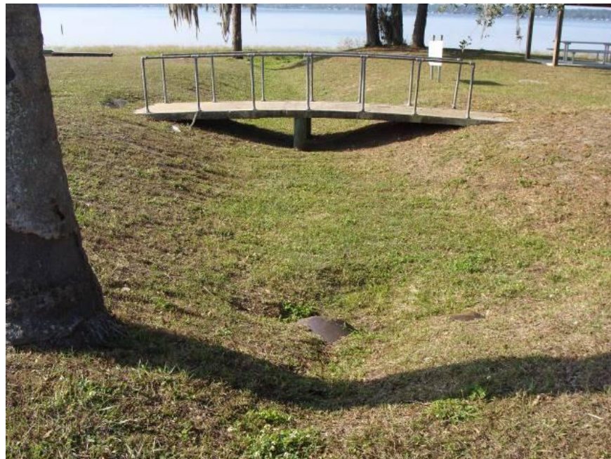
FIGURE 21: CAMP BLANDING CAMPGROUND SWALE FROM AVENUE A TO KINGSLEY LAKE
