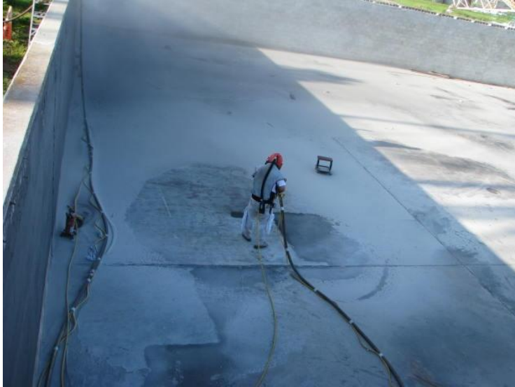
SANDBLASTING INSIDE THE SOUTH TANK BEING CONVERTED TO THE CHLORINE CONTACT TANK
