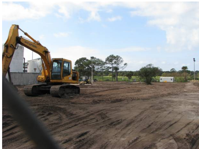
FIGURE 13: BACKFILL OF JACKSONVILLE BEACH OLD WWTP AREA
