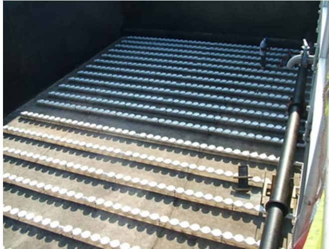
NEW FINE BUBBLE DIFFUSERS ALLOW FOR BETTER OXYGEN TRANSFER
