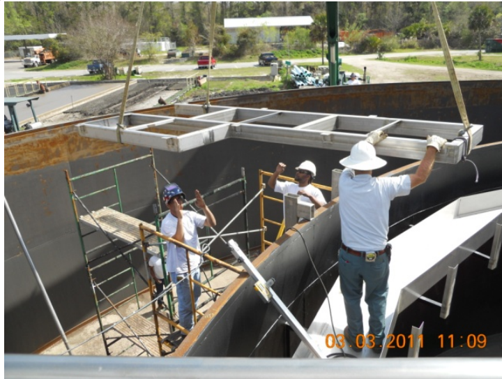
ASH STREET WWTF STAINLESS STEEL BRIDGEWORK FOR INVERT MIXER-AERATORS DURING PHASE 2 CONVERSION
