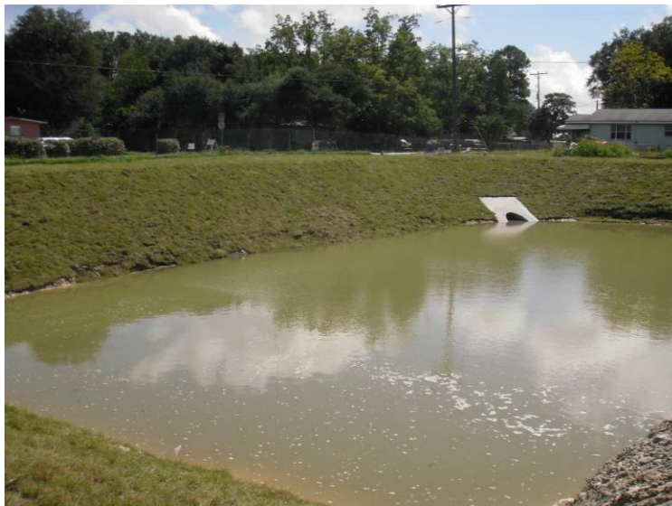
FIGURE 29: CITY OF JACKSONVILLE PINE FOREST/LARSEN ACRES POND CONSTRUCTION
