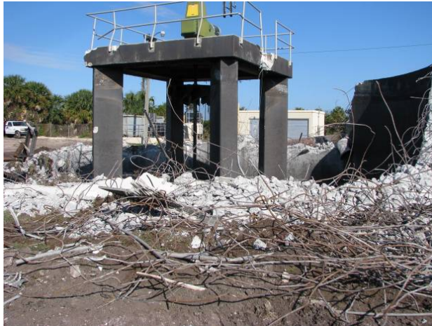
FIGURE 12: JACKSONVILLE BEACH WWTP DEMOLITION OF THE OLD PLANT TANKS
