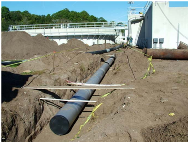
REPLACED DETERIORATED CAST IRON AIR PIPING WITH STAINLESS STEEL PIPE
