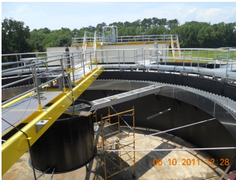
ASH STREET WWTF CLARIFIER #2 UNDER CONSTRUCTION
