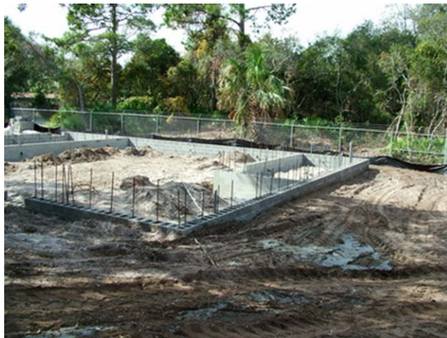
CONSTRUCTING NEW SLUDGE TREATMENT BUILDING WITH CENTRIFUGE
