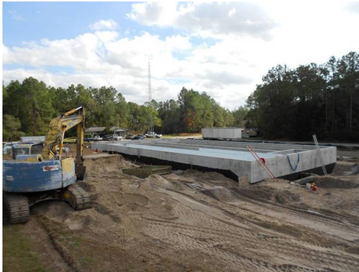
FIGURE 6: PALATKA WWTF UPGRADES
