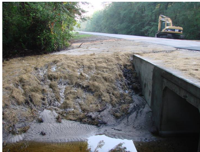
NORTH FORK BLACK CREEK DURING CULVERT REPLACEMENT
