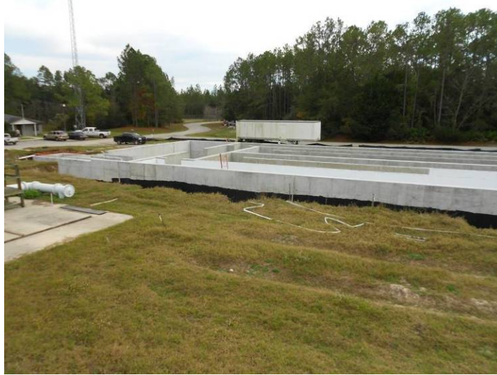
FIGURE 5: PALATKA WWTF UPGRADES
