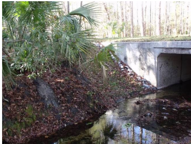
FIGURE 39: CAMP BLANDING NORTH FORK BLACK CREEK AFTER INSTALLATION
