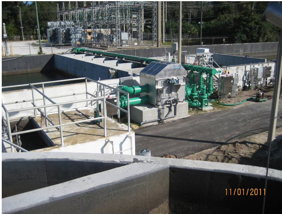
NEPTUNE BEACH UPGRADED WWTf
