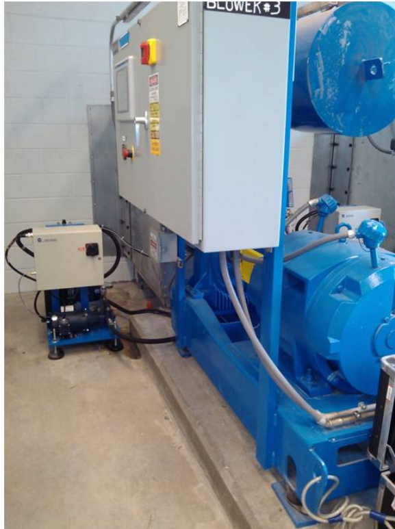
FIGURE 8: CITY OF ATLANTIC BEACH WWTP FOUR NEW, EFFICIENT BLOWERS REPLACED NINE EXISTING BLOWERS
