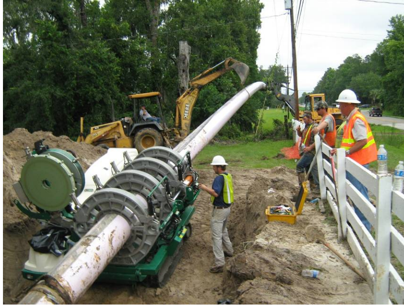
FIGURE 10: CCUA FUSING 18-INCH RECLAIMED WATER MAIN FOR DIRECTIONAL DRILL INSTALLATION ON COUNTY ROAD 209
