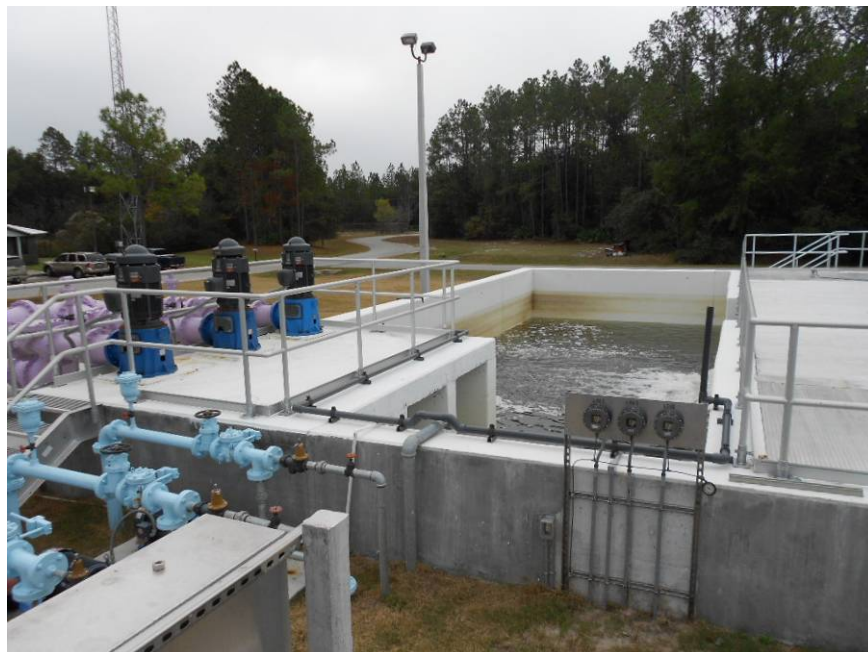
CITY OF PALATKA WWTP UPGRADES
