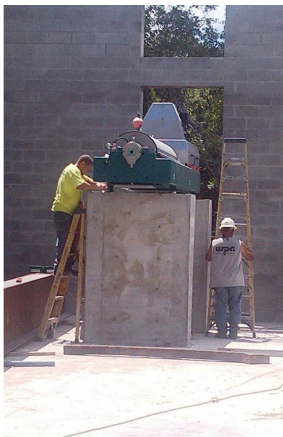
NEW CENTRIFUGE INSTALLED TO REPLACE INEFFICIENT SLUDGE DRYING BEDS
