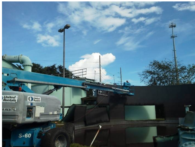
TANKAGE AND EQUIPMENT AT WWTP #2 DEMOLISHED AND THE PLANT PROPERLY ABANDONED
