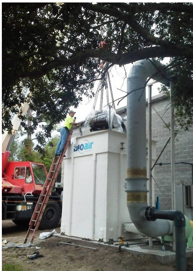
ODOR CONTROL EQUIPMENT INSTALLED
