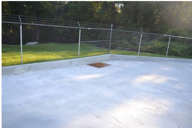
FIGURE 24: CAMP BLANDING WWTP NEW EROSION CONTROL STRUCTURE
