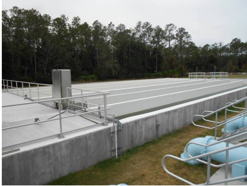
FIGURE 3: CITY OF PALATKA WWTP NEW CONTACT CHAMBER
