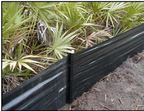
A properly installed silt fence can prevent sediments from migrating off site.
