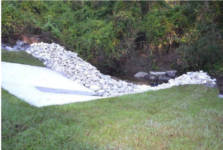
FIGURE 25: CAMP BLANDING WWTP NEW EROSION CONTROL STRUCTURE
