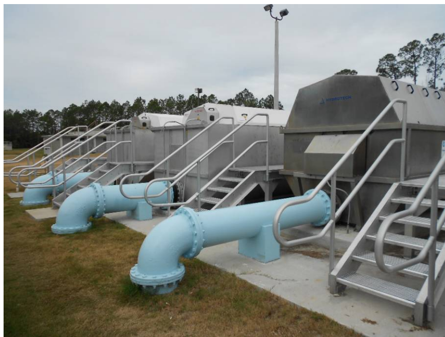
CITY OF PALATKA WWTP UPGRADES
