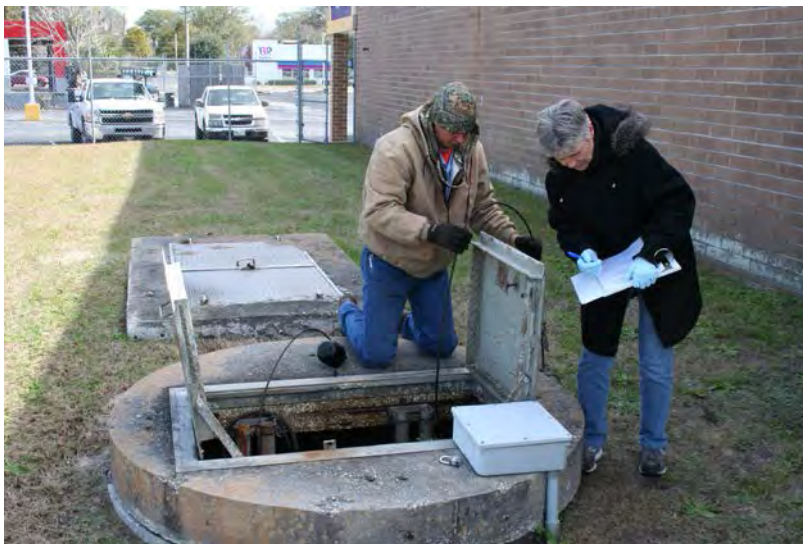
FIGURE 13: COJ EQD STAFF CONDUCTS INSPECTION OF SEWAGE LIFT STATION IN THE BIG FISHWEIR WATERSHED
