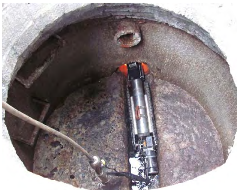
FIGURE 20: NS MAYPORT VIDEO INSPECTION OF A SEWER LINE
