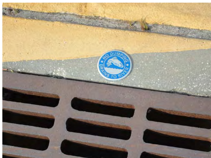
FIGURE 22: NS MAYPORT STORM DRAIN MARKER
