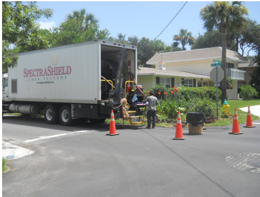
FIGURE 18: CITY OF ATLANTIC BEACH MANHOLE REHABILITATION PROJECT
