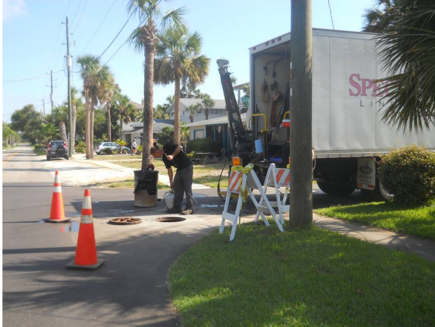
FIGURE 17: CITY OF ATLANTIC BEACH MANHOLE REHABILITATION PROJECT
