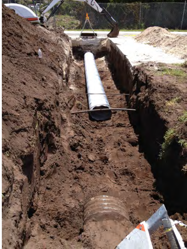
FIGURE 19: CITY OF NEPTUNE BEACH STORM SEWER REPAIRS ON 5 TH STREET
