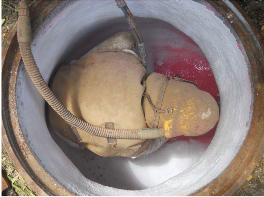
FIGURE 21: CITY OF ATLANTIC BEACH APPLICATION OF SPECIALTY COATING ON REHABILITATED MANHOLE
