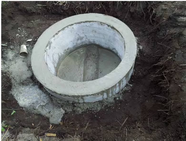
FIGURE 20: CITY OF NEPTUNE BEACH SANITARY SEWER REHABILITATION ON FOREST AVENUE
