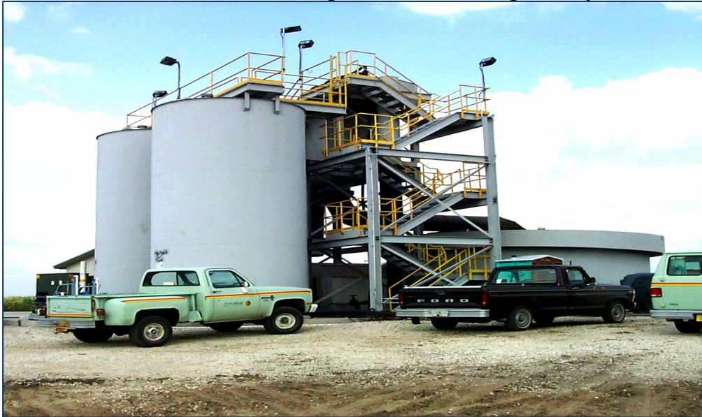
Figure 2 Lake Hollingsworth Dewatering Facility
