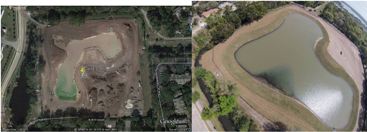
FIGURE 12: SEMINOLE COUNTY CASSEL CREEK RSF IN CONSTRUCTION
