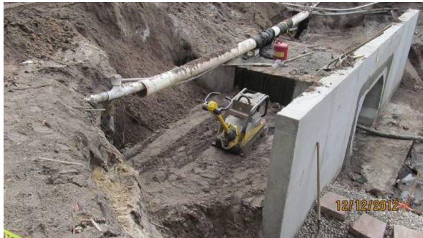
FIGURE 5: CITY OF LONGWOOD FAIRY LAKE OUTFALL UNDER CONSTRUCTION
