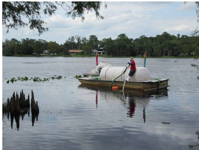
FIGURE 2: CITY OF CASSELBERRY QUEENS MIRROR LAKE ALUM TREATMENT IN SEPTEMBER 2012
