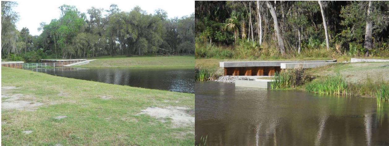
FIGURE 11: CITY OF WINTER SPRINGS SOLARY CANAL PROJECT INFLOW (LEFT) AND OUTFLOW (RIGHT)
