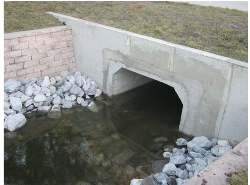
Longwood Fairy Lake Outfall
