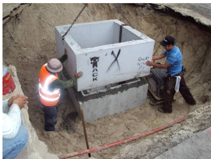
CITY OF MAITLAND LAKE MAITLAND BASIN DRAINAGE IMPROVEMENTS
