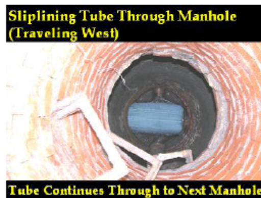
Sliplined Pipe in Manhole
