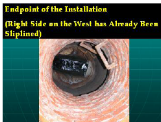
Finished Pipe in Manhole
