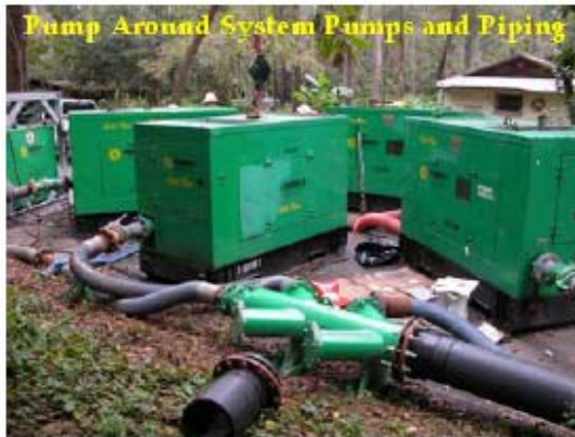
Figure H-9. Installation sequence of a Hogtown Creek sliplining project Pump Around (Hogtown Creek Basin)
