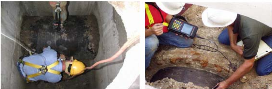
Figure H-11. GRU engineers and crews performing pipe wall thickness testing
