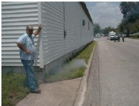
Illegal Connections to GRU Wastewater Collection System: Apartment Rain Gutter
