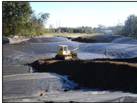
Depot Park Phase 1 stormwater pond under construction
