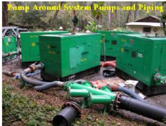
Figure H-9. Installation sequence of a Hogtown Creek sliplining project Pump Around (Hogtown Creek Basin)
