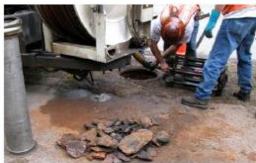
Tuberculation Removed in Pipeline Preparation with Hydraulic Chain Cutter
