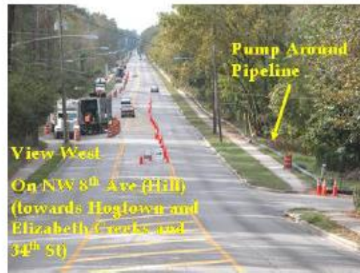
Figure H-9. Installation sequence of a Hogtown Creek sliplining project Pump Around (Hogtown Creek Basin)
