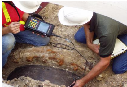
Figure 3.10. GRU engineers and crews performing pipe wall thickness testing
