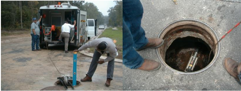
Figure 3.4. GRU closed-circuit TV inspection unit
