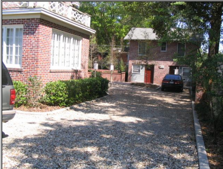
Figure 3.14. Pervious driveway into the Heritage Oaks Condominium Complex in Gainesville
