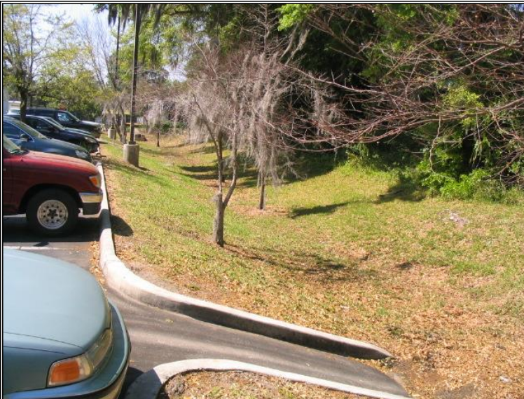
Figure 3.13a. Vegetated swale around the Walgreens Pharmacy on NW 13 th Street, Gainesville
