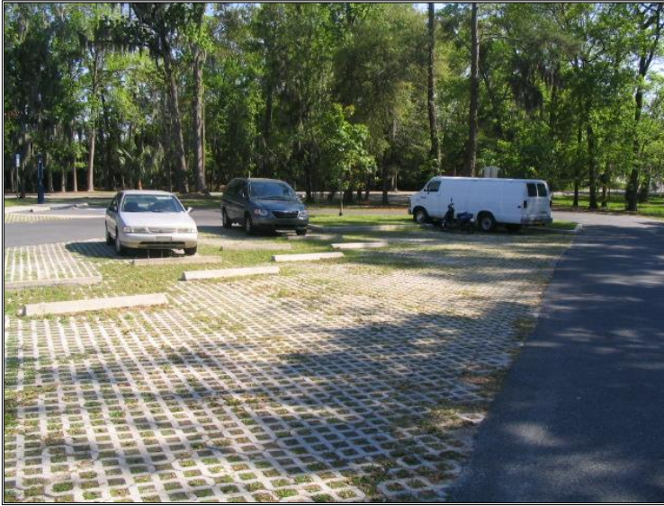
Figure 3.15. Permeable pavement at the UF Bat House parking lot
