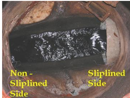
Figure 3.9. Sliplined major gravity mains adjacent to Hogtown Creek and tributaries
