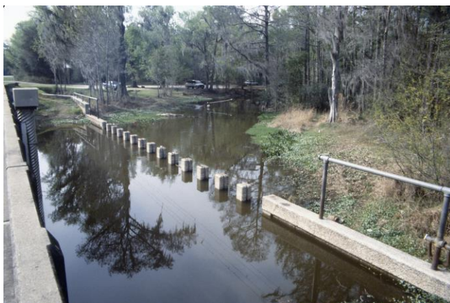
Figure 2.5. Photograph of former weir at the outlet of Newnans Lake, SR 20 Bridge, January 1992
