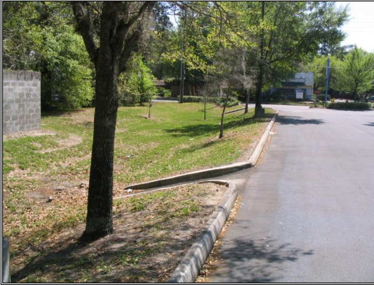
Figure 3.13b. Vegetated swale around the Walgreens Pharmacy on NW 13 th Street, Gainesville
