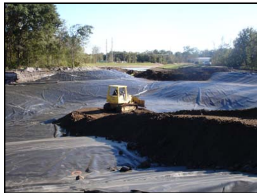
Depot Park Phase 1 stormwater pond under construction
