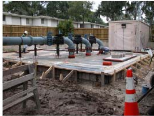
Renovated Receiving Manhole, Wetwell, Drywell and Completed Lift Station
