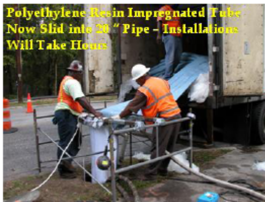
Polyethylene Resin Impregnated Tube Now Slid into 20" Pipe - Installations Will Take Hours
