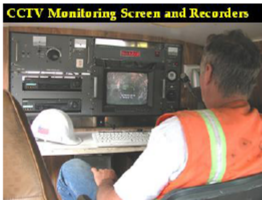
CCTV Monitoring Screen and Recorders
