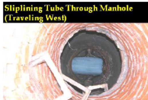
Sliplining Tube Through Manhole (Traveling West)
