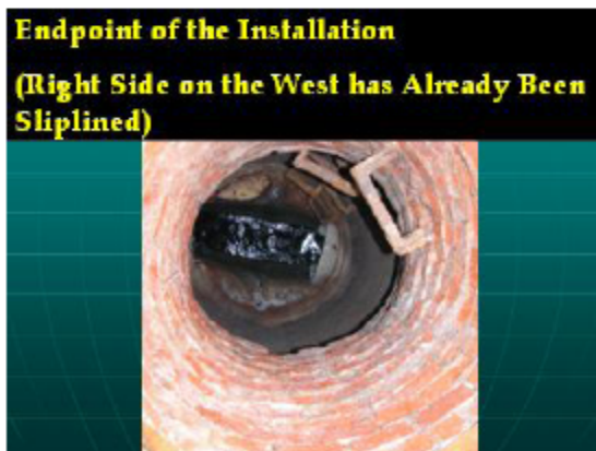
Figure __ Shows GRU sliplined major gravity mains adjacent to Hogtown Creek and its tributaries since 1994.
