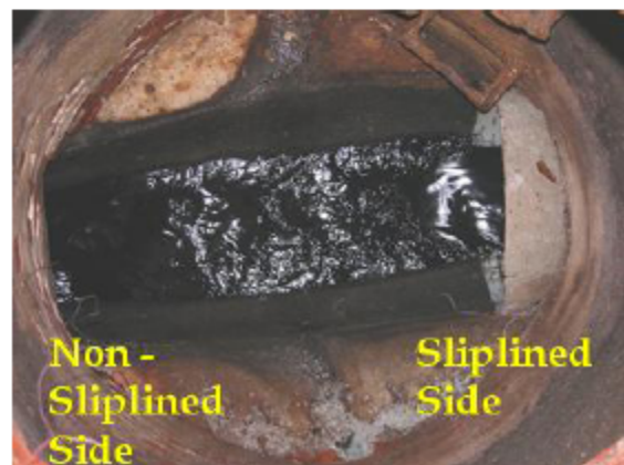
Figure __ Shows GRU sliplined major gravity mains adjacent to Hogtown Creek and its tributaries since 1994.
