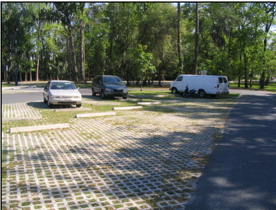
Figure 39. Permeable pavement at the University of Florida Bat House parking lot
