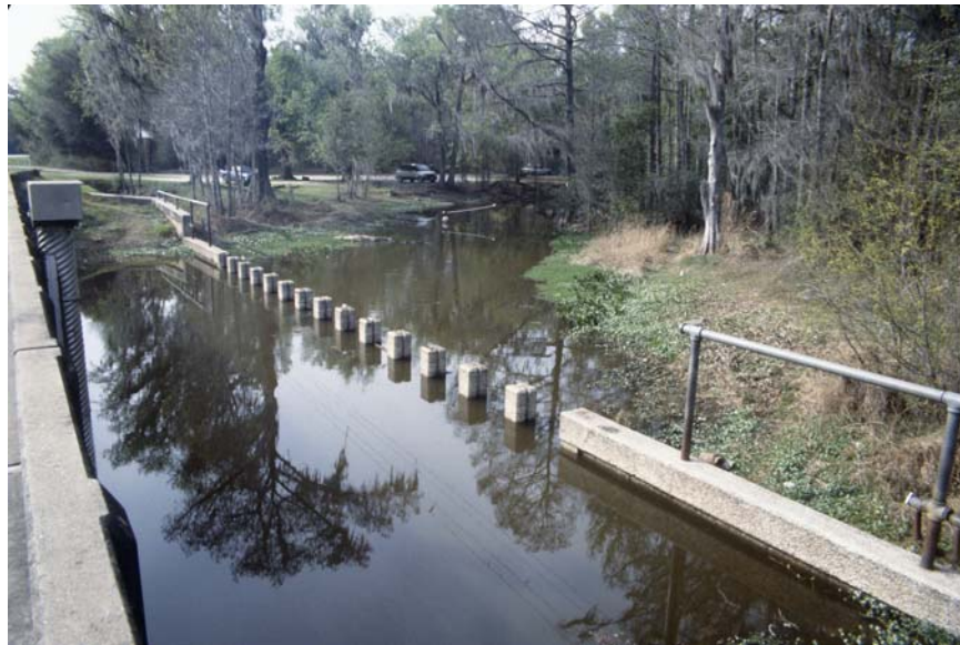
FIGURE 15. PHOTOGRAPH OF FORMER WEIR AT THE OUTLET OF NEWNANS LAKE, STATE ROAD 20 BRIDGE, JANUARY 1992
