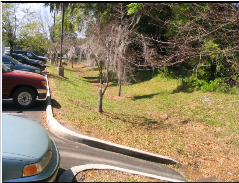
Figure 38. Vegetated swales around the Walgreens Pharmacy on NW 13 th Street, Gainesville, FL
