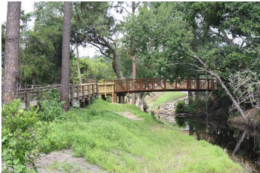
FIGURE 3: ESCAMBIA COUNTY’S JONES CREEK EAST STREAM RESTORATION PROJECT
