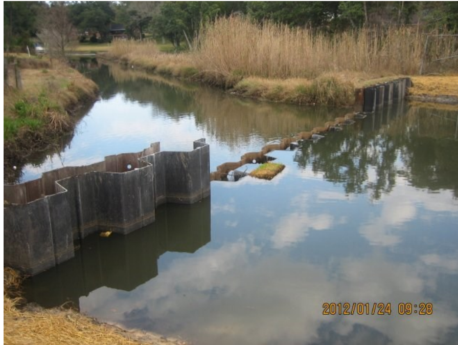
FIGURE 6: ESCAMBIA COUNTY’S “W” STREET SEDIMENTATION BASIN
