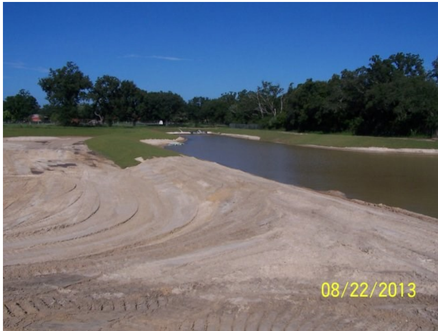
FIGURE 4: ESCAMBIA COUNTY’S LEXINGTON TERRACE STORMWATER RETROFIT PROJECT
