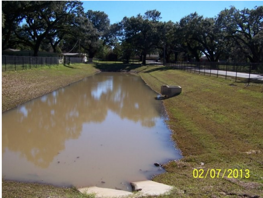
FIGURE 2: ESCAMBIA COUNTY’S AVERY STREET DRAINAGE IMPROVEMENTS PROJECT
