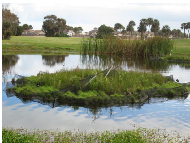
d. Netting collapsed near end of project.
