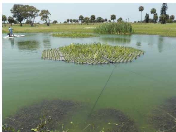
c. Mats attached to shoreline using rope
