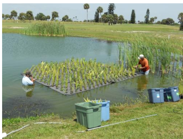
c. Mats attached together to create desired size
