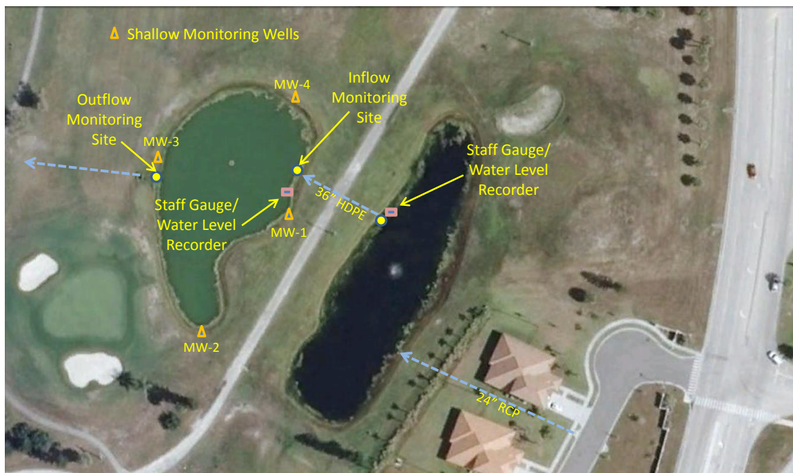
Figure 4. Field Monitoring Equipment Installed at the PAFB Pond Site.
