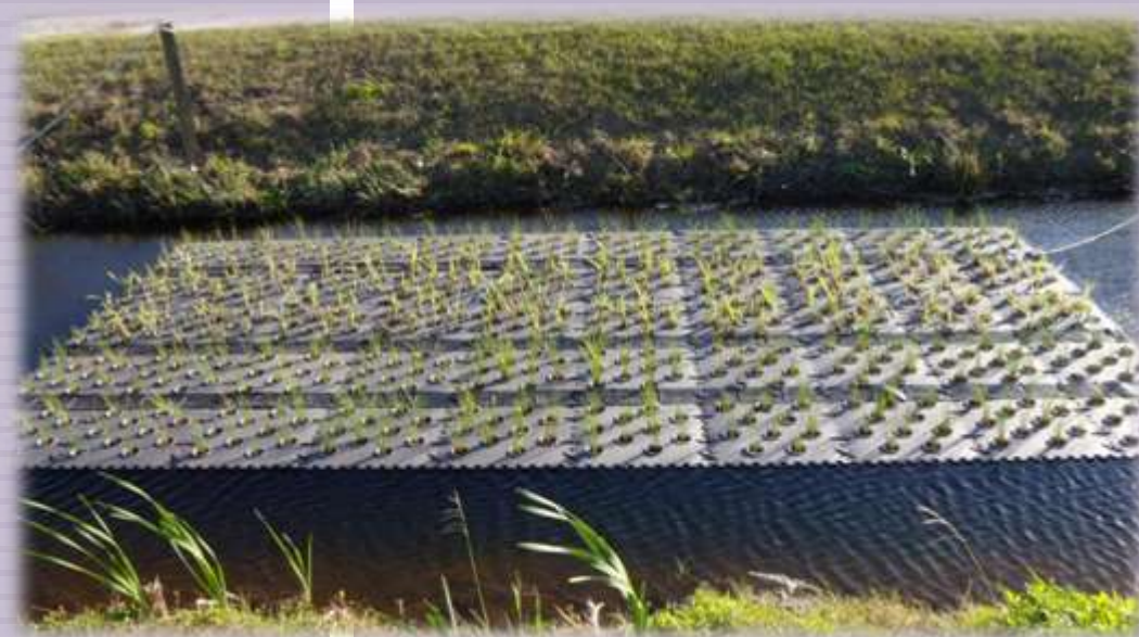
Mats as first installed in ditch.
