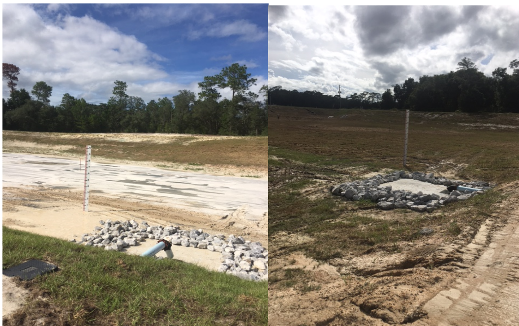
(a) BAM RIB looking northeast
