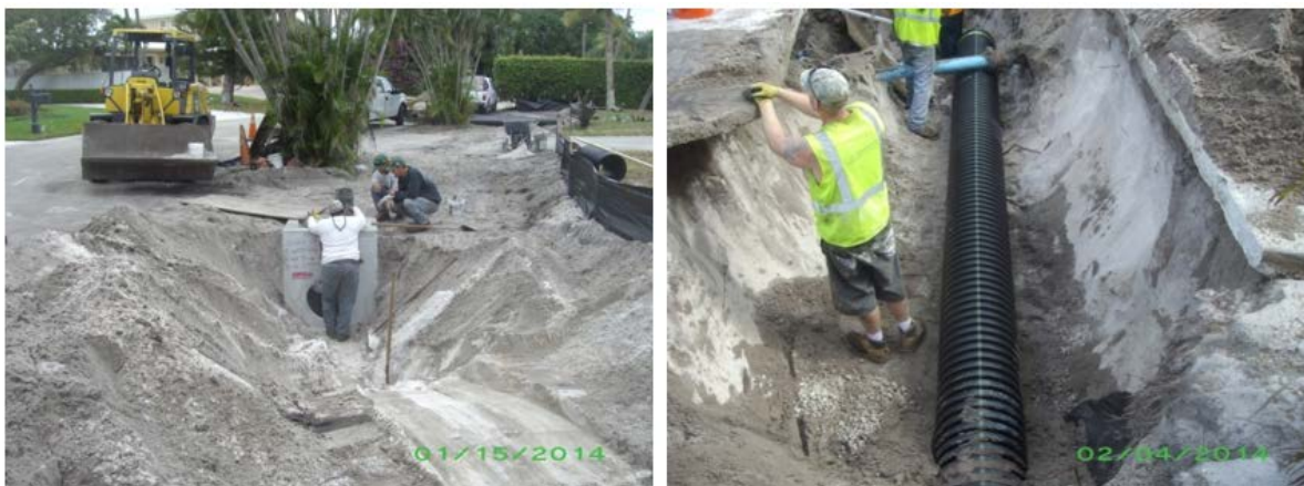
FIGURE 7: TOWN OF SEWALL'S POINT HIGH POINT EXFILTRATION PROJECT UNDER CONSTRUCTION
