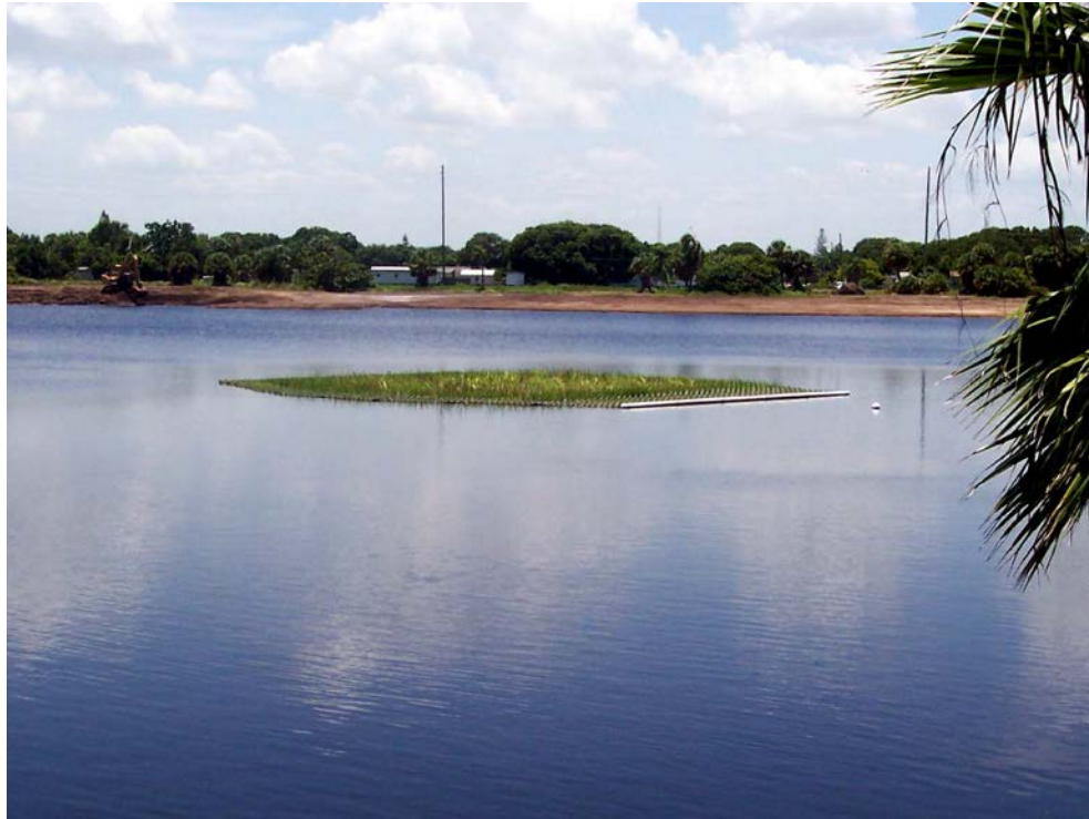
Indian Hills Recreation Area Stormwater Improvements - First Floating Island Installed - 06/26/14
