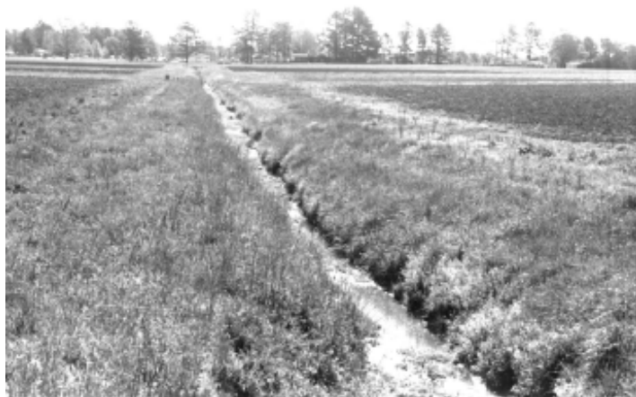
Figure 8. Surface drainage system.
