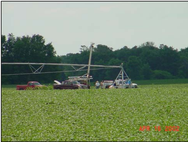
Figure 9 April 16, 2002. Repair crew on sight restoring the electrical wiring of the irrigation system.
