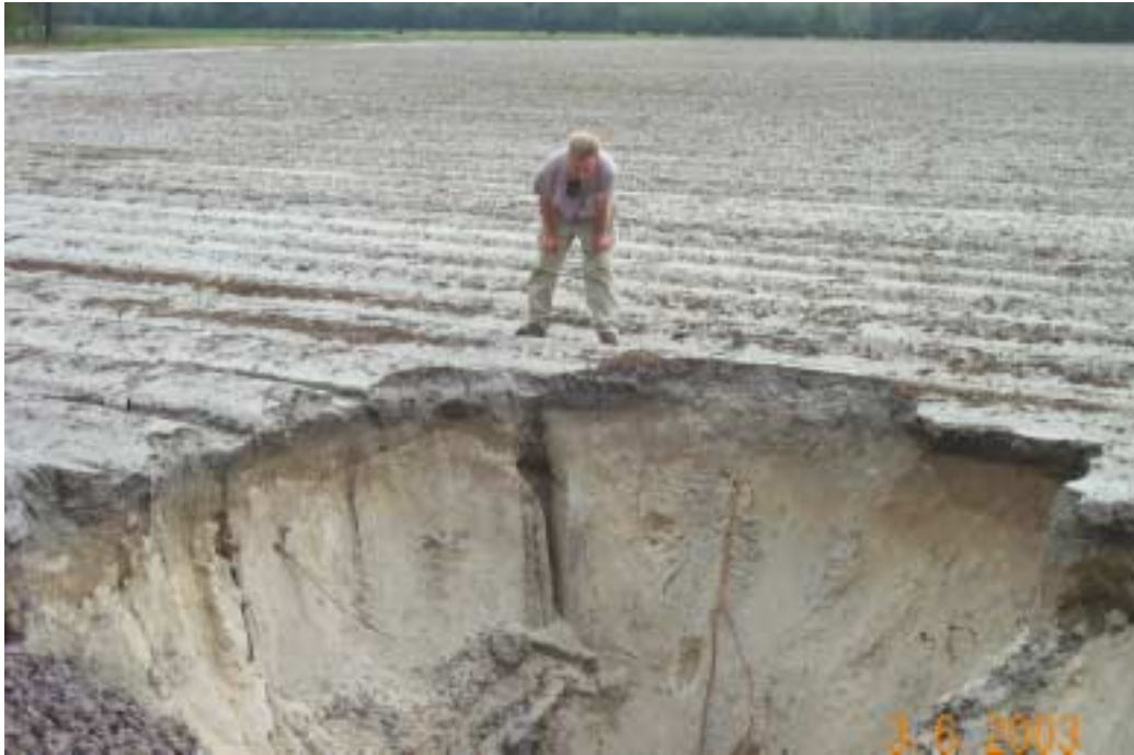
Figure 45. An example of a sinkhole that opened in the demonstration field during the course of the project. Also note the open channels that were exposed by the sinkhole.
