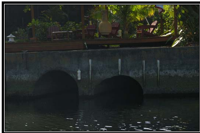
Photograph 32. There are several significant stormwater outfalls, such as this double culvert, that line the main channel of the Lower Hillsborough River. These conveyance systems are potential sources of fecal pollution to the tributary.
