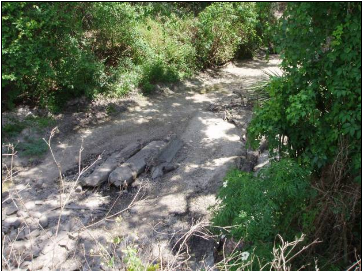
Figure 64. Main branch of Turkey Creek is completely dry at SR 60 during follow up visit [04/09/12]. All upstream portions inspected that day appeared in similar conditions.
