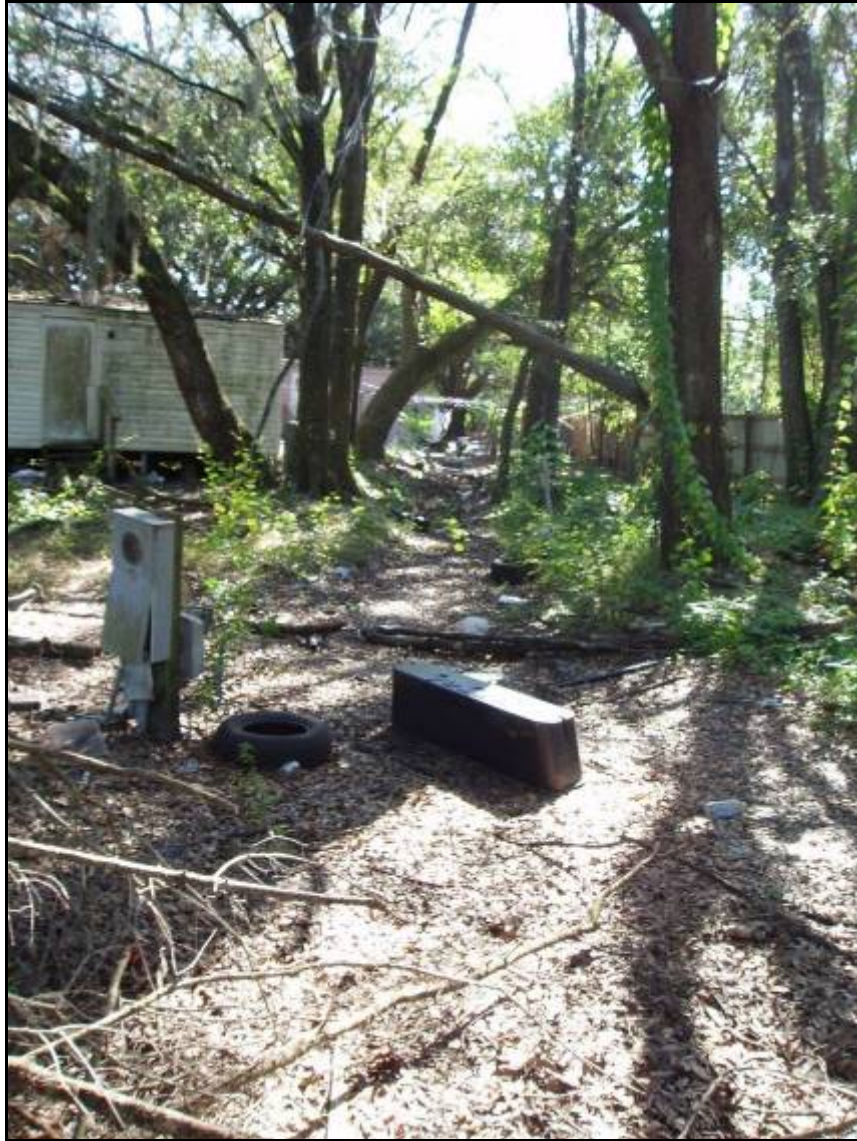
Figure 46. Conveyance in Starlite MHP containing considerable amounts of trash.
