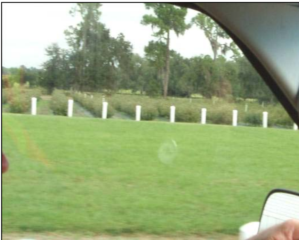
Figure 13. Septic system drain field serving migrant housing on Higgins Farm. The drain field is cordoned off and appears well functioning.
