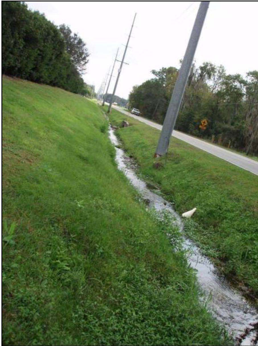
Figure 18. Ditch downstream of Walden Lakes outfall [east on Trapnell]. Water flows to the cross drain where it joins the easternmost tributary of Turkey Creek.
