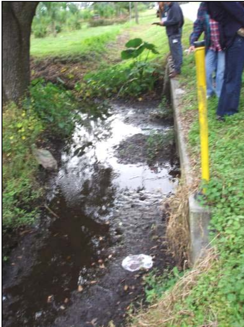
Figure 8. Convergence of several ditches and a cross drain running under Sydney Dover Rd south of Walden Sheffield Rd. Oily sheen, wildlife tracks, and litter visible in the creek. Spoke with adjacent landowner, George Williamson Farm, regarding hydrology and water quality. George Williamson Farm participates in the FDACS BMP enrollment program.
