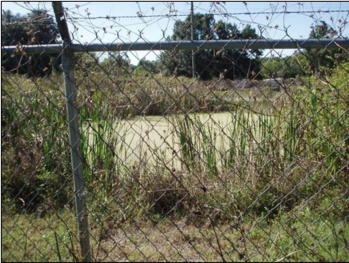
Figure 49. Treated effluent from Starlite MHP's OSTDS is discharged to this pond. Overall, the pond and conveyance systems are overgrown and contain considerable amounts of trash and sediment, possibly contributing to bacterial growth.
