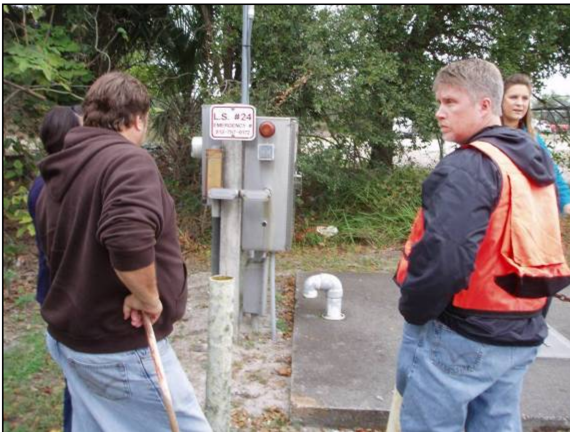
Figure 15. Lift station 24 operated by the City of Plant City. No history of discharge and appears to be functioning appropriately. Emergency number is posted, and notification light appears operational. Additionally, all lift stations in the Turkey Creek watershed are inspected weekly and equipped with telemetry notification.
