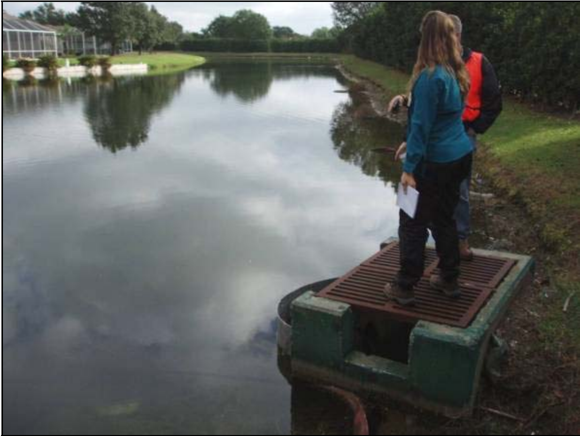
Figure 17. Wet detention pond in Walden Lakes subdivision. Control structure discharges directly to the outfall pictured in Figure 16.
