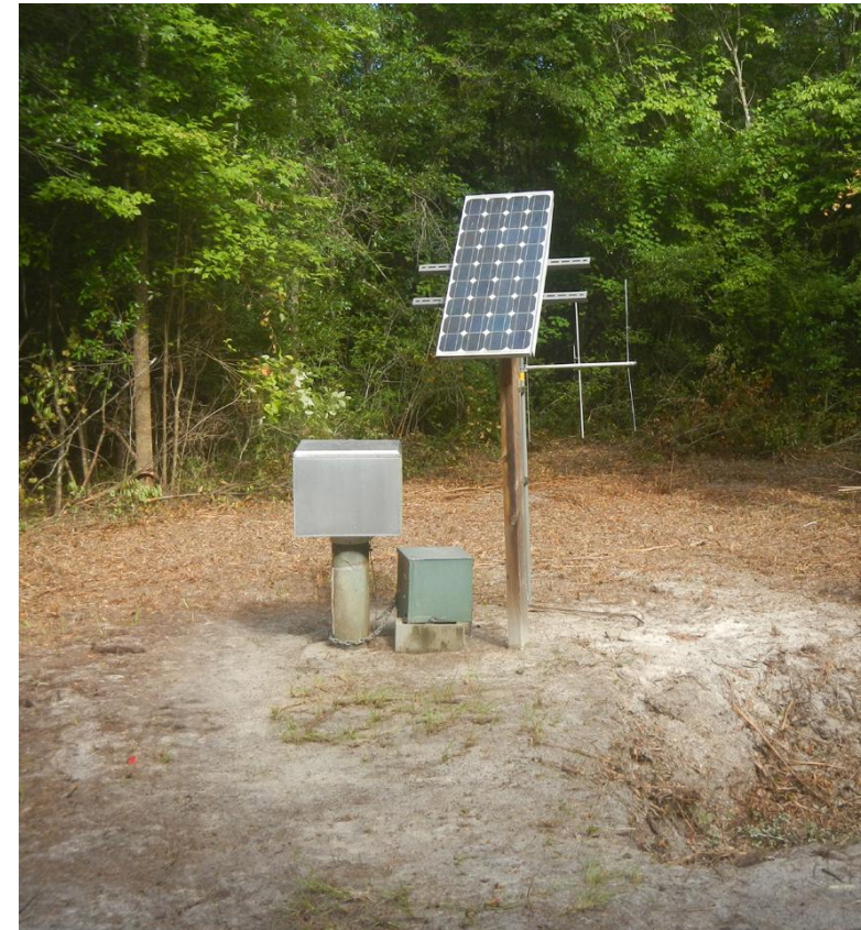
Well #3: K- and A/K-Tunnel access
