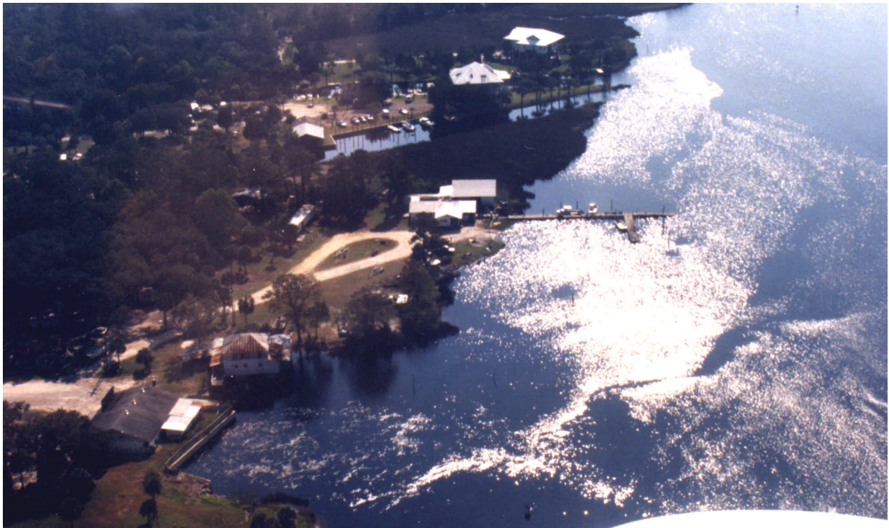
Figure 14. Aerial photograph of Spring 1, view downstream, October 1998. Spring boil shows as circular sun-glitter directly to the right of the straight bulkhead in the lower left. Magnitude of the spring's discharge is indicated by its semi-circular slick, which extends half-way across the picture. FGS photograph.
