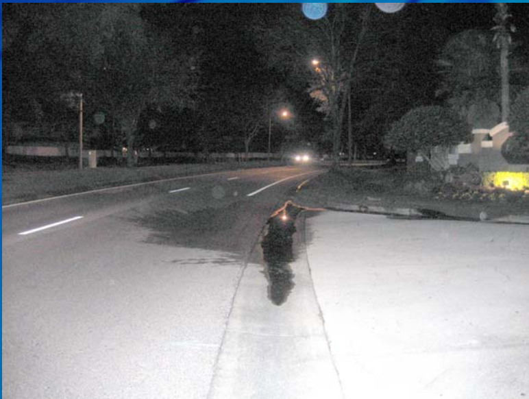
Reuse Accumulates in Gutters
